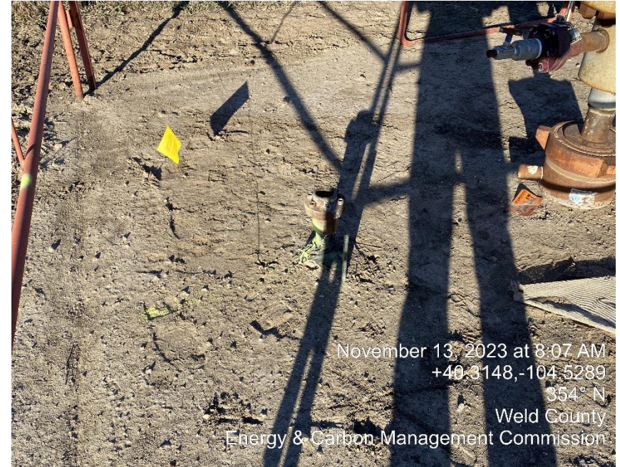
Riser is not identified and no OOSLAT tag visible or LO/TO.
