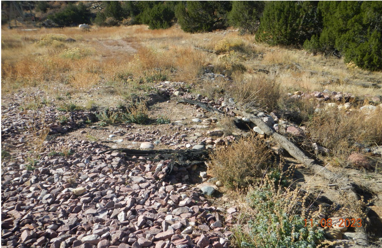
Photo 2. Facing toward the drainage crossing which has been washed out and has not been repaired. Previous corrective action was not completed.
