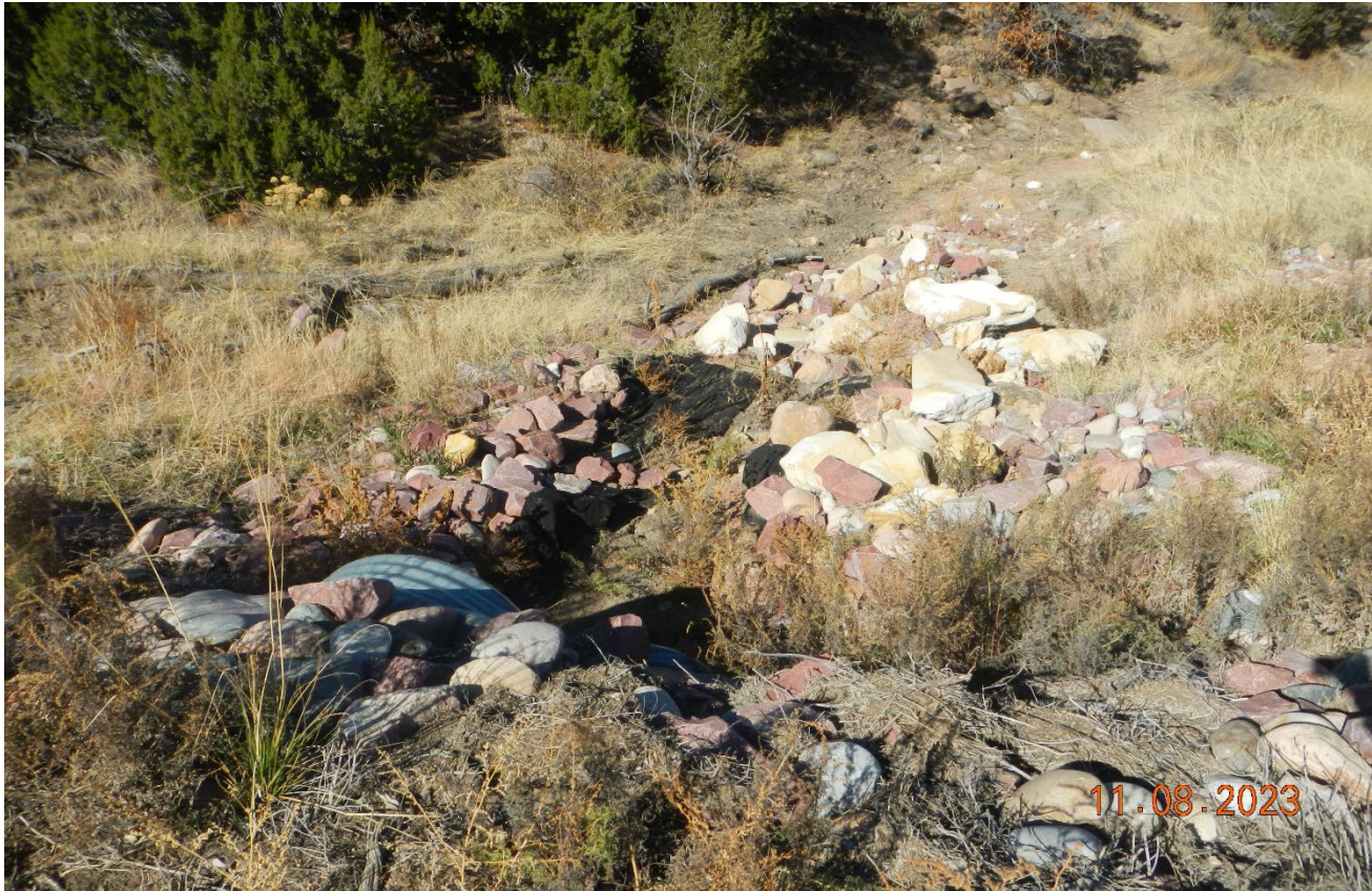
Photo 3. View of culvert outlet shows displaced rock. Outlet protection will need to be reinstalled. Previous corrective action was not completed.
