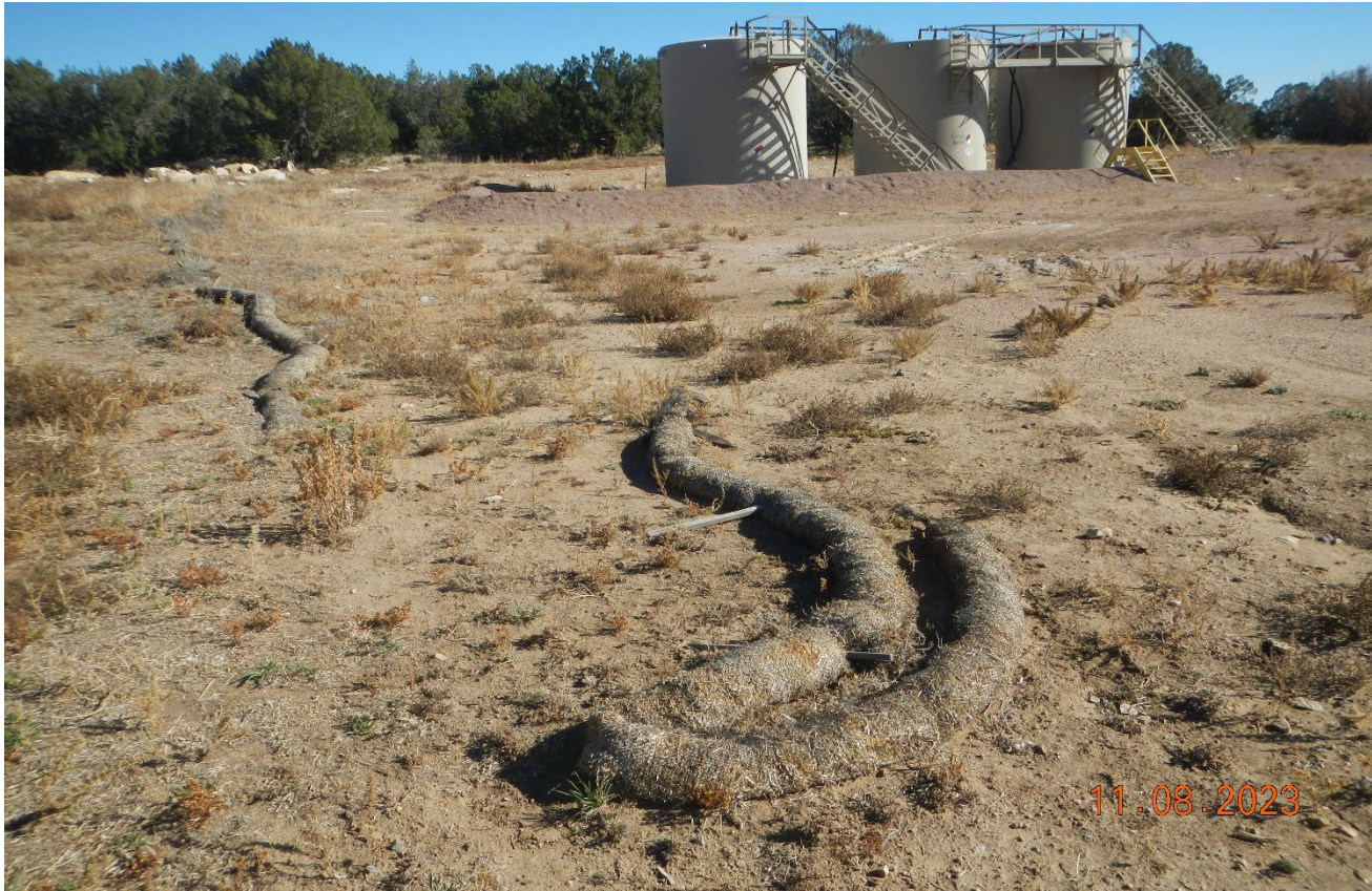
Photo 5. Facing north toward the location. There are displaced wattles that need to be repaired. Previous corrective action was not completed.
