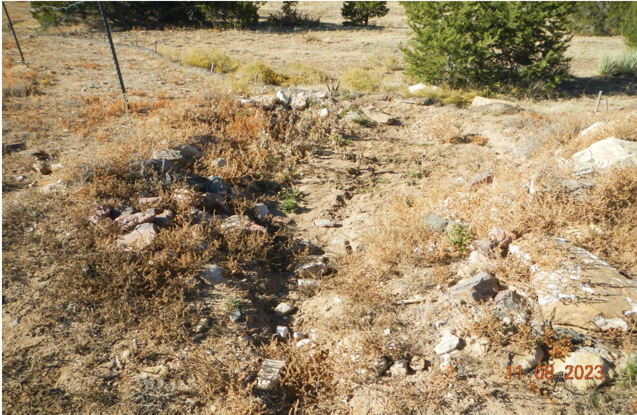
Photo 6. The sediment trap at the west side of the location is filled in with sediment.
