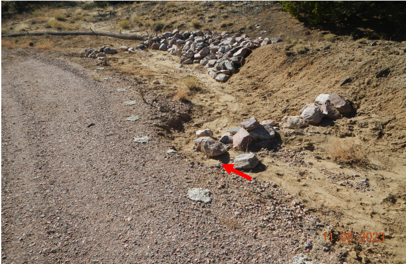
Photo 2. There are several check dams that are in need of maintenance. Red arrow points to where stormwater is eroding around the check dam.
