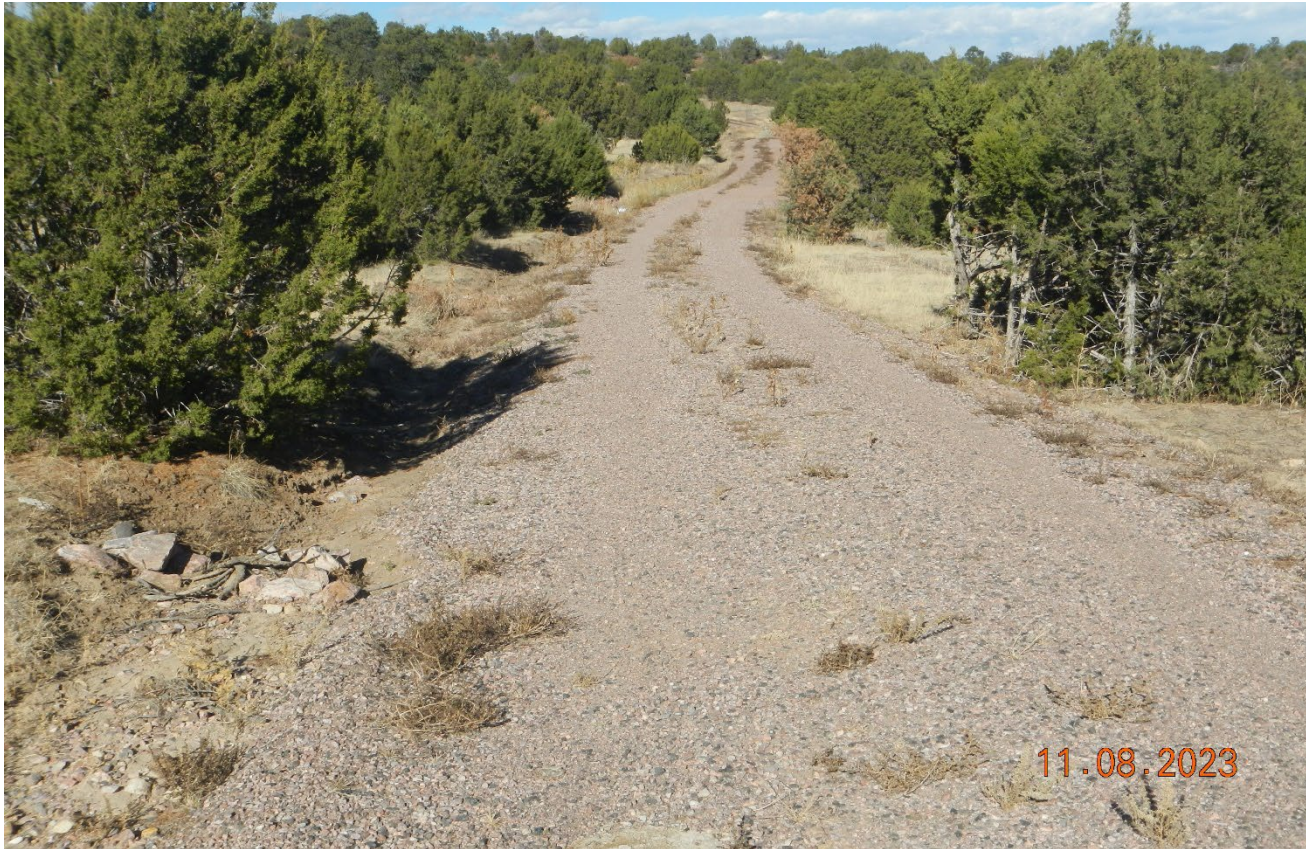
Photo 1. Facing northwest along the access road. There are some check dams where stormwater is going around the check dam. BMP maintenance is needed.
