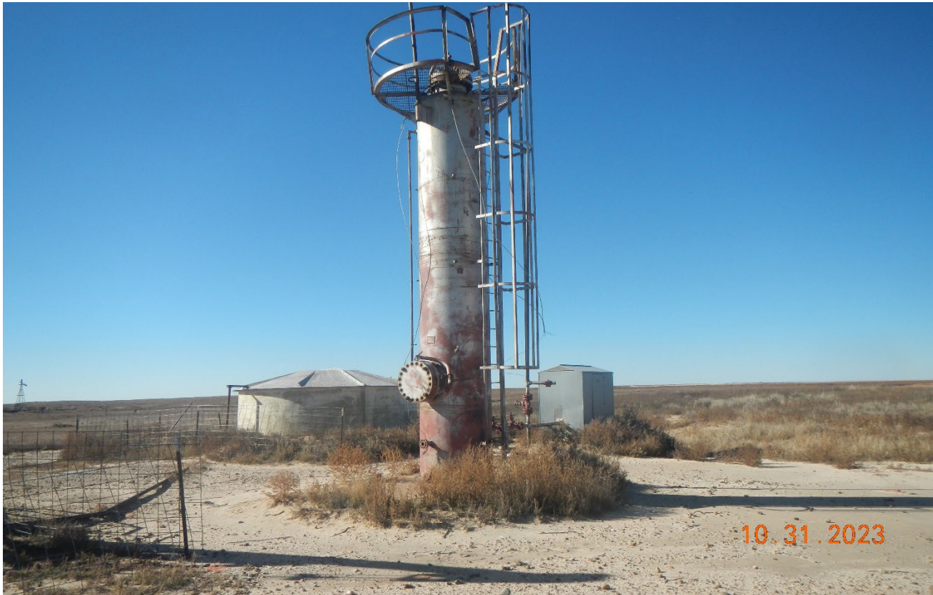
Photo 5. Facing toward the separator. There is no containment around the separator.
