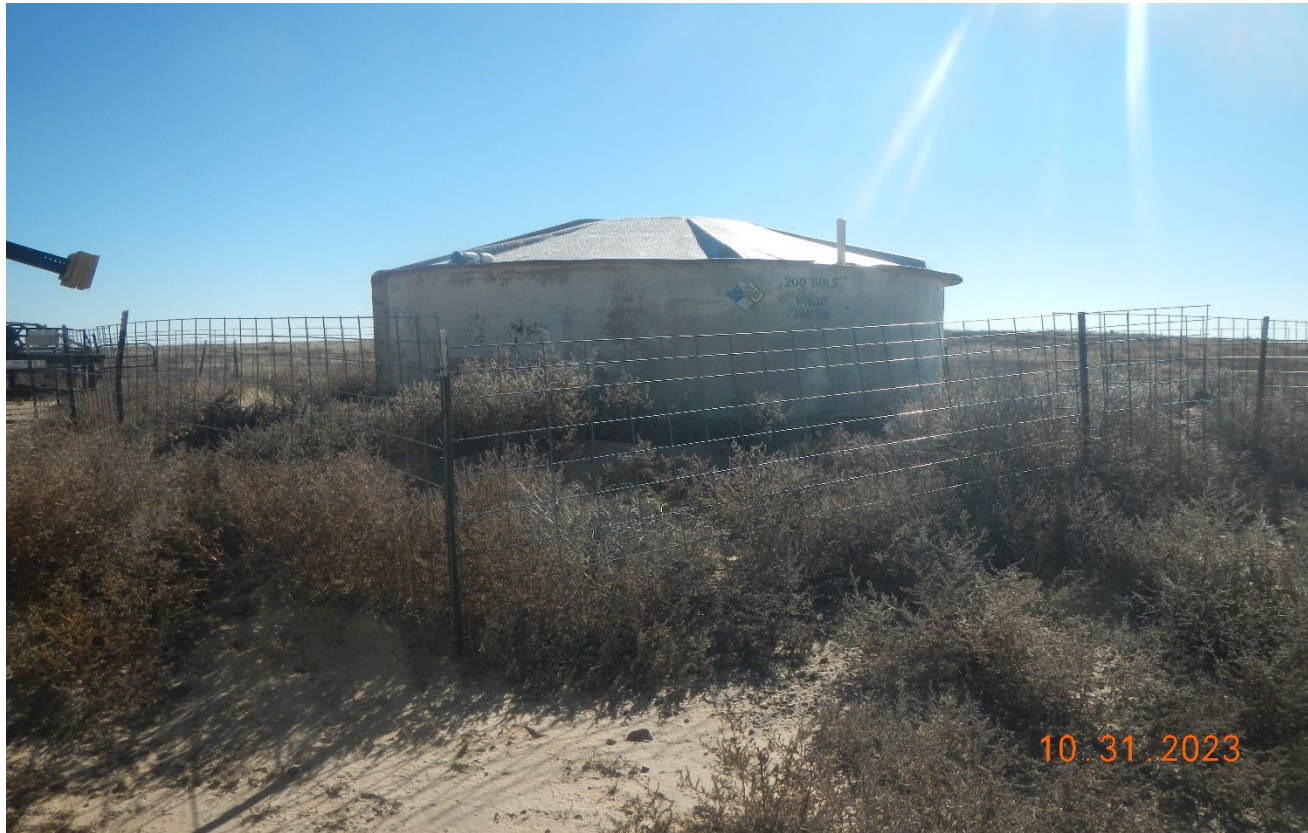
Photo 5. Facing toward the tank. There are weeds around the tank that are a fire hazard. Secondary containment is insufficient. And the labeling is faded.
