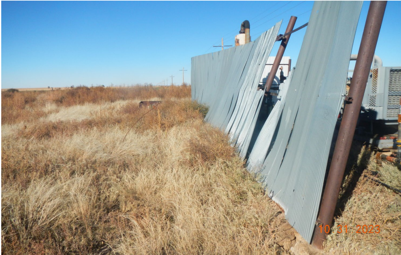
Photo 3. The wall behind the compressor engine is leaning over about to fall down.
