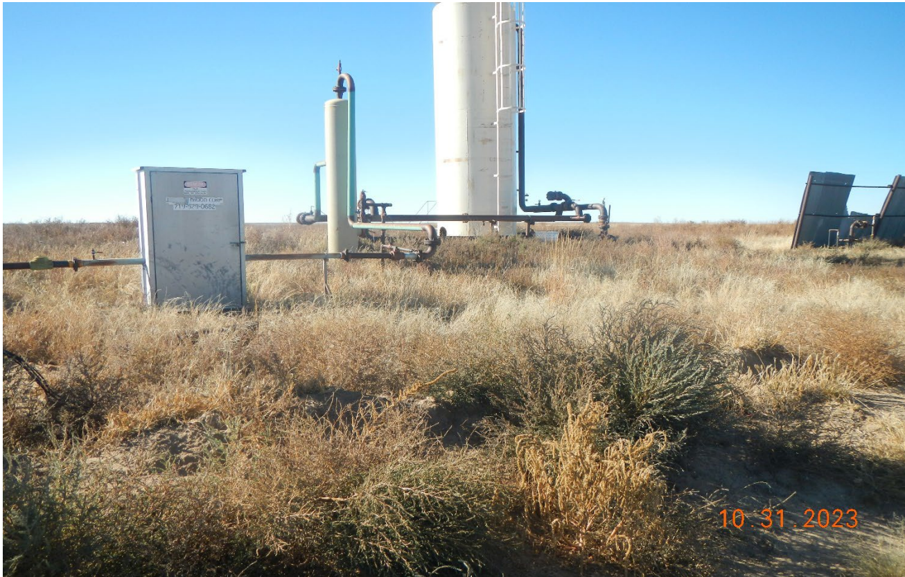
Photo 1. Facing west toward the Walsh/Bishop Gas Compressor. There is weeds and dry vegetation around the equipment which is a fire hazard.
