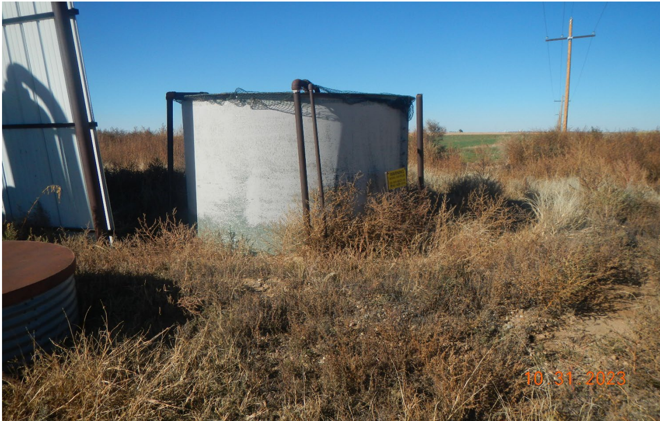
Photo 6. There are weeds around the open top tank and insufficient secondary containment.
