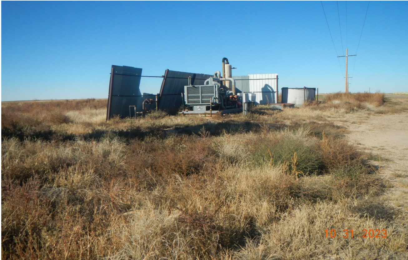
Photo 2. Facing northwest toward the Walsh/Bishop Gas Compressor. There is weeds and dry vegetation around the equipment which is a fire hazard.
