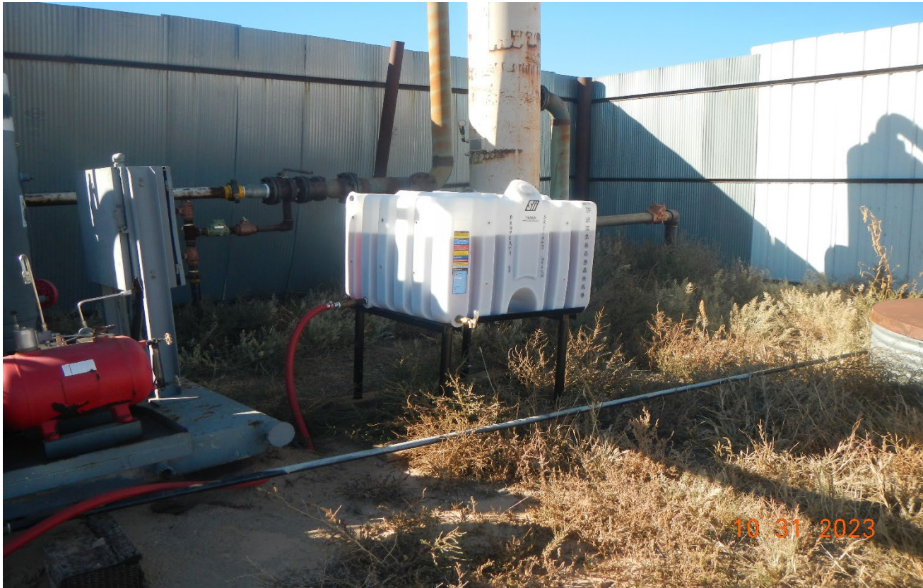
Photo 5. There is no secondary containment at the chemical tote.
