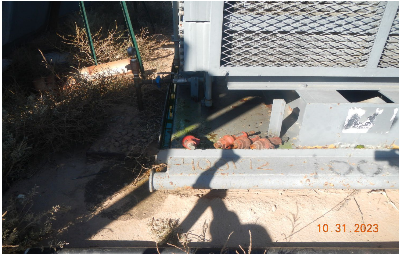
Photo 4. There is green liquid glycol I the engine skid that must be cleaned up.
