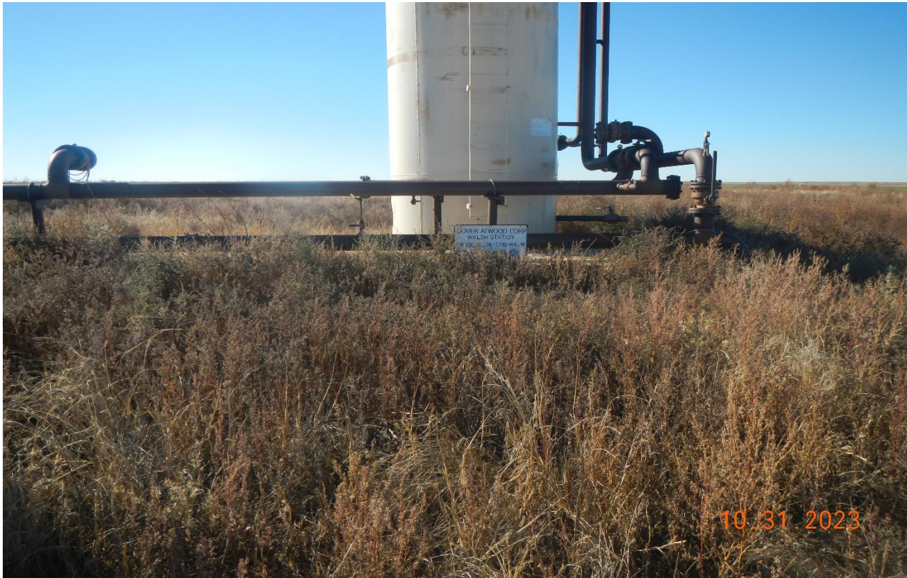
Photo 8. Facing toward the separator. There is no secondary containment and the location sign is obscured by weed cover.
