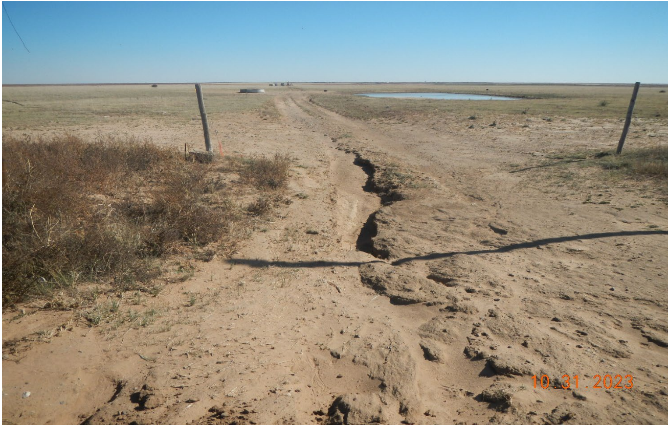
Photo 1. Facing east at the access road. There is erosion along the road that needs to be repaired and stabilized..
