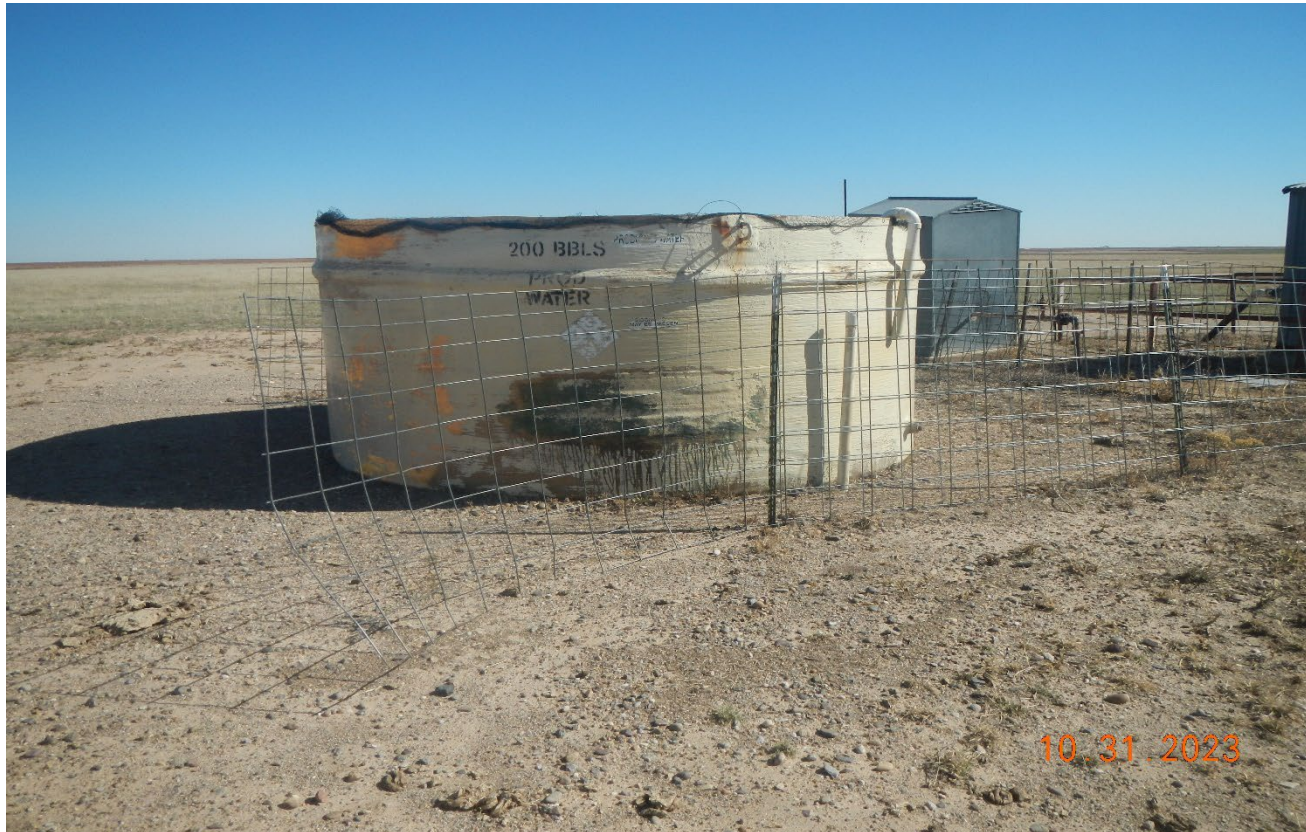
Photo 4. There is no secondary containment around the open top tank. The fence around the equipment is in disrepair.
