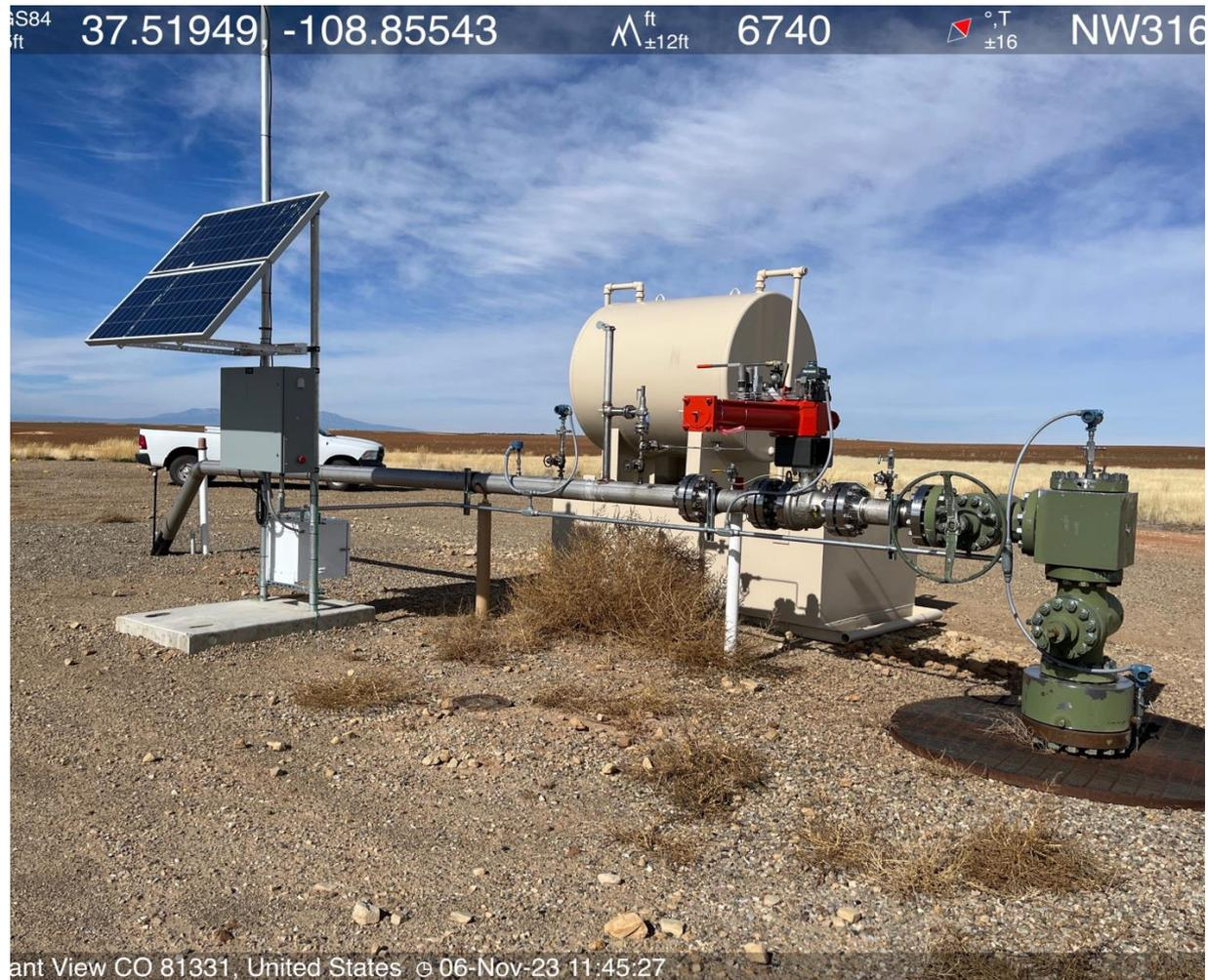
**Photo #5 View of the wellhead, flowline, and ancillary equipment.**
