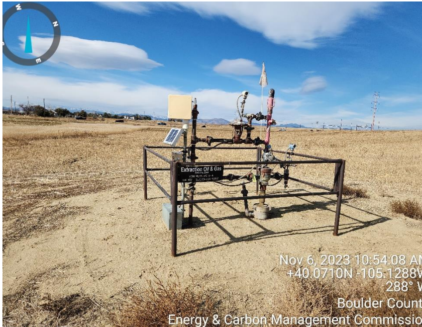
Photo 1 well head and equipment
