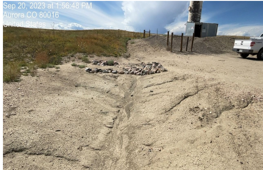
Photo 3. Photo of erosion from stormwater along tank battery south side. Photo taken facing west.
