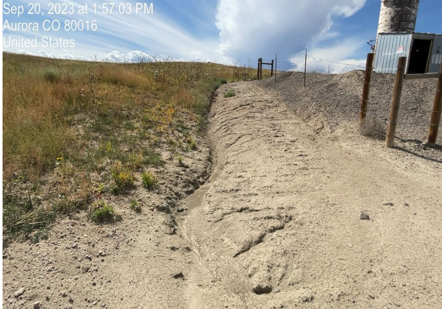
Photo 5. Photo of erosion from stormwater along tank battery south side, and weeds (kochia & russian thistle) . Photo taken facing west.
