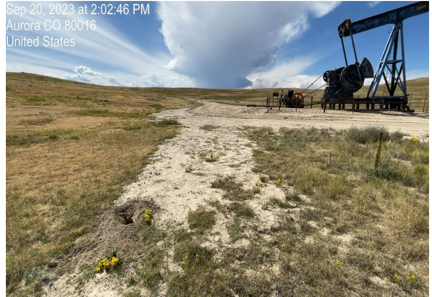
Photo 12. Photo of erosion from stormwater leaving well pad onto adjacent lands. Photo taken facing west.
