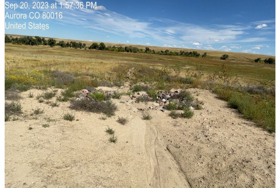
Photo 6. Photo of check dam filled with sediment from stormwater erosion along tank battery south side. Sediment observed leaving location. Photo taken facing east.
