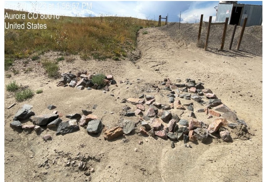
Photo 4. Photo of check dam filled with sediment from stormwater erosion along tank battery south side. Photo taken facing west.
