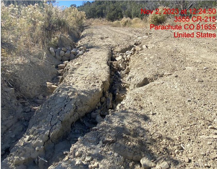
Insufficient Erosion Controls on Access Road – Photo #07334
