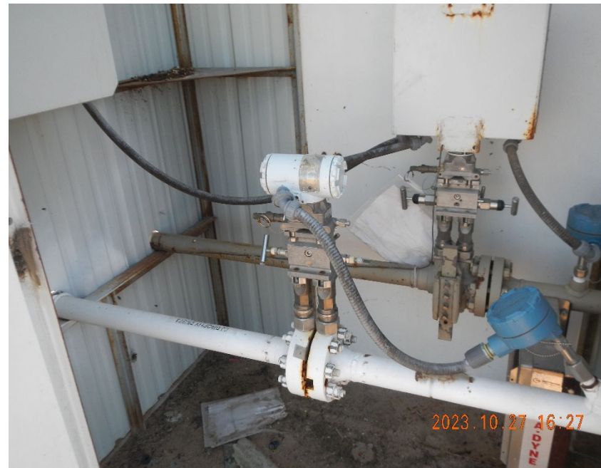
4. Digital gas meter. Calibration log needs to be replaced.
