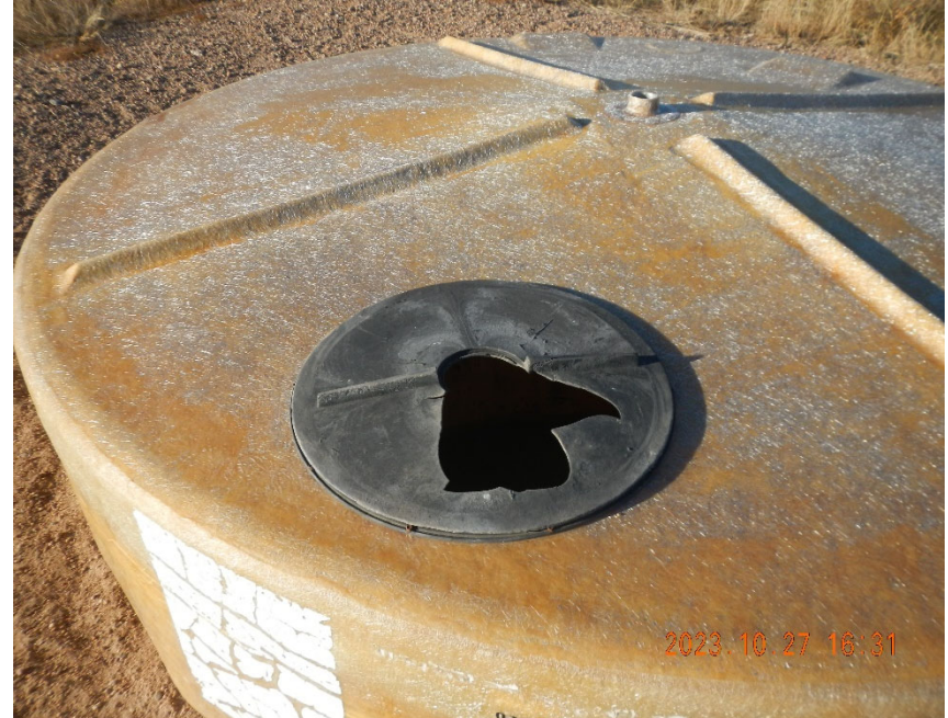
6. Produced water tank broken hatch cover.
