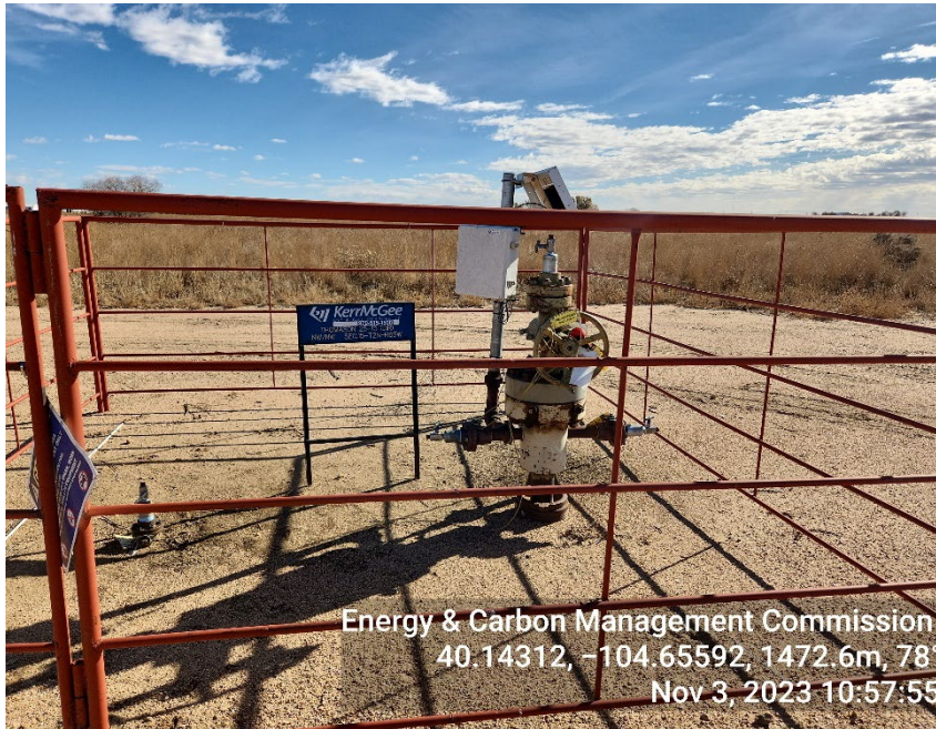
Photo 3: TA Wellhead
