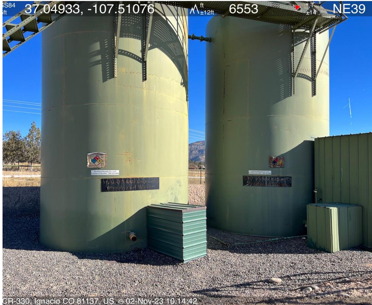
Photo #6 View of not legible contents/volume labels and NFPA placards.
