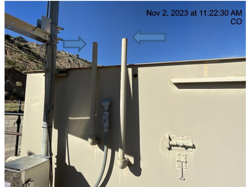
Photo # 5169 PRV & Rupture disc vent lines lack caps
