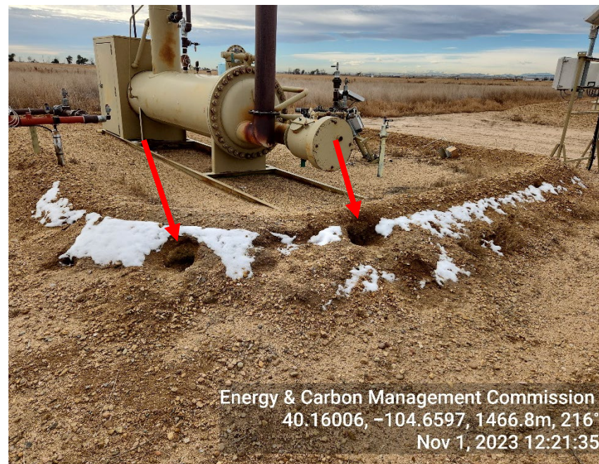
Photo 8: Damaged earth berm
