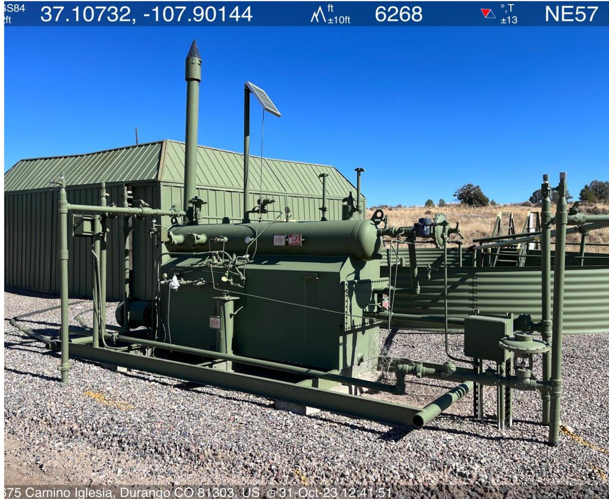
Photo #5 View of separator/dehydrator.
