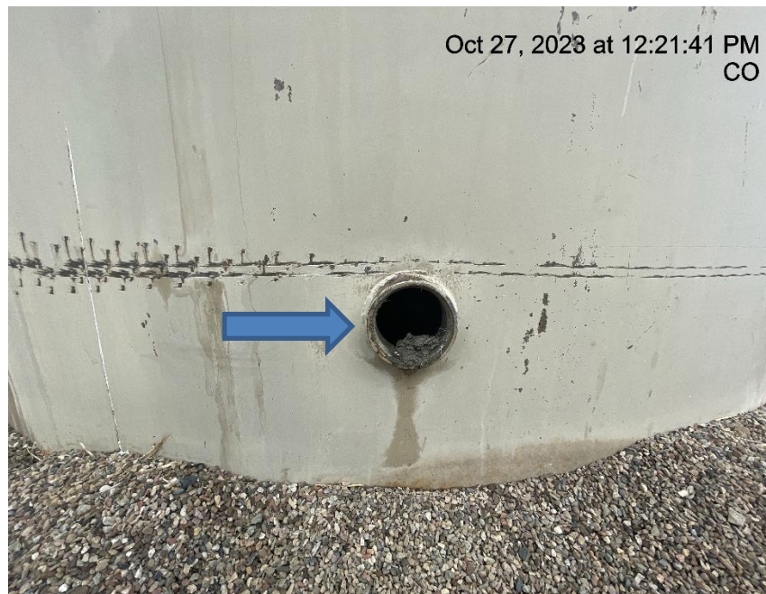
Photo # 4577 Open ended port on production tank/wildlife hazard
