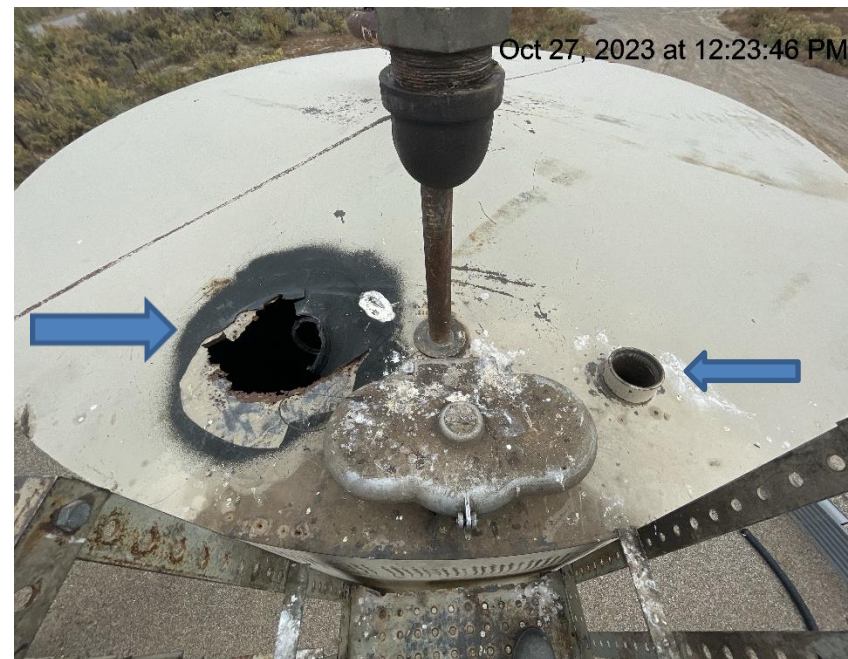
Photo # 4578 Corrosion & hole in top of production/open ended port/wildlife hazards
