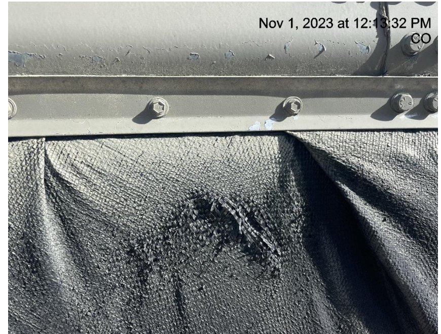
Photo # 4993 Hole in liner/liner needs maintenance
