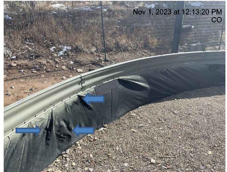
Photo # 4991 Holes in liner/liner needs maintenance
