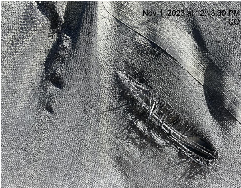
Photo # 4992 Holes in liner/liner needs maintenance
