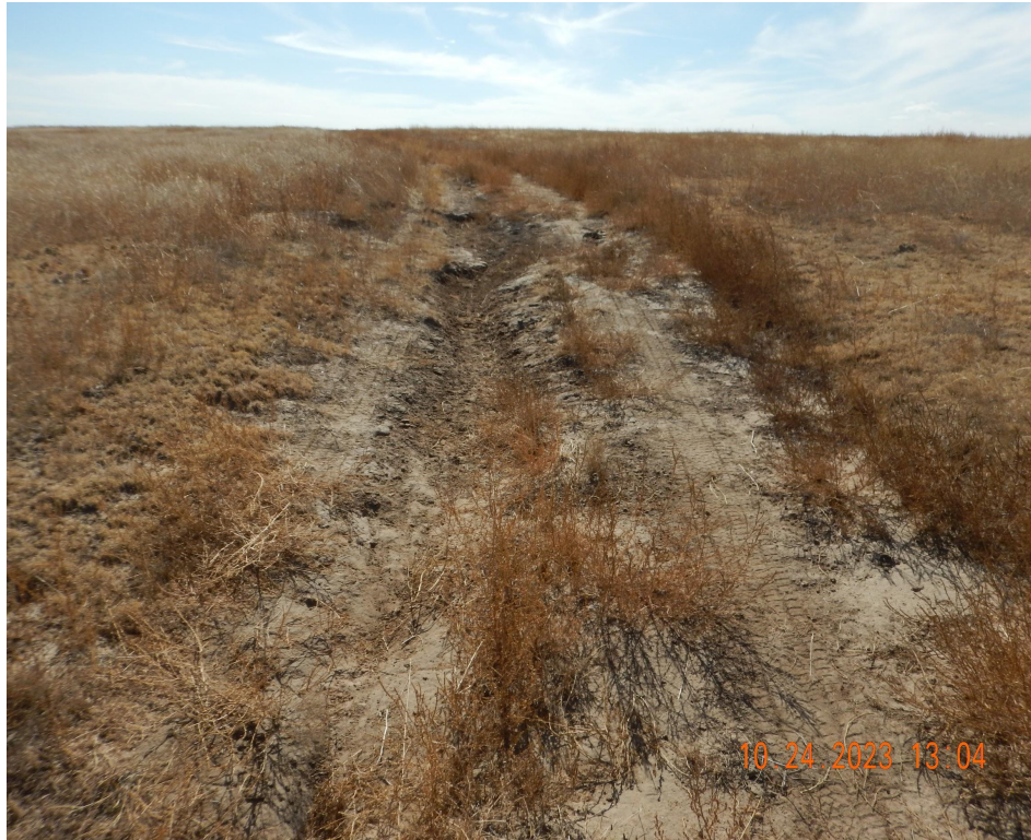
Photo 1. Photo taken from a portion of the access road ~225' south of the southern location, facing South. Photo illustrates the access road has not been reclaimed, erosion is evident, and unmanaged weeds (kochia and russian thistle) observed along the access road.
