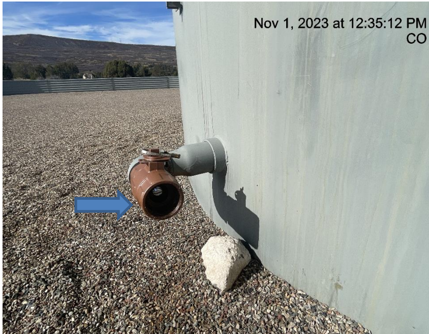
Photo # 5024 Open ended load line
