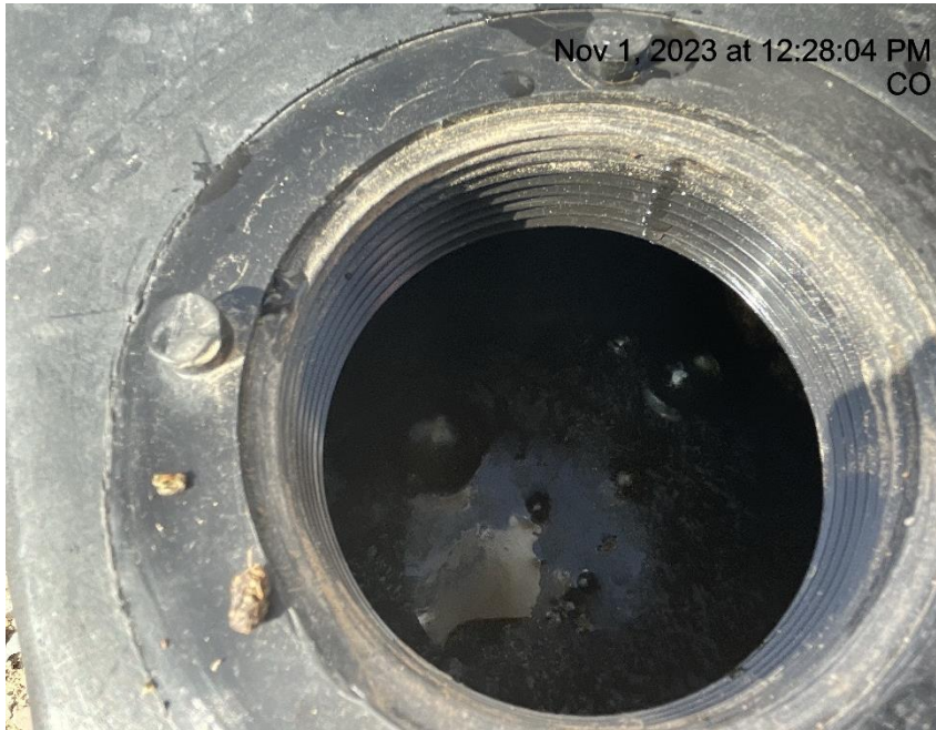
Photo # 5025 Failure to maintain chemical BMP/chemical tank containment full of fluid.
