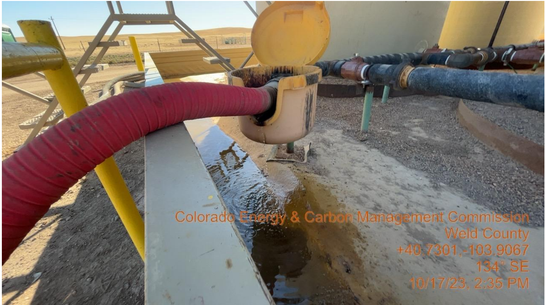
Photo 2. The photo was taken at the East end of the tank batteries facing Southeast. The photo illustrates produced water actively spilling into secondary containment.
