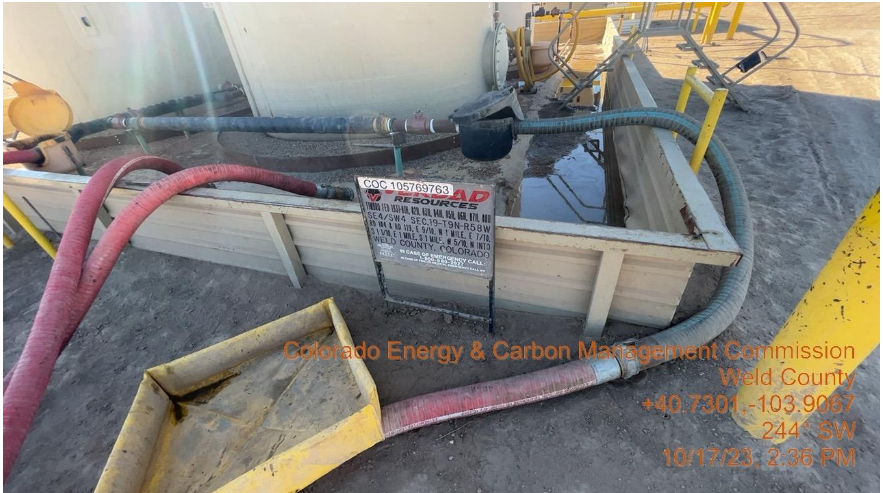
Photo 1. The photo was taken of the location sign. Photo illustrates produced water spilled into secondary containment as well as hoses outside secondary containment.
