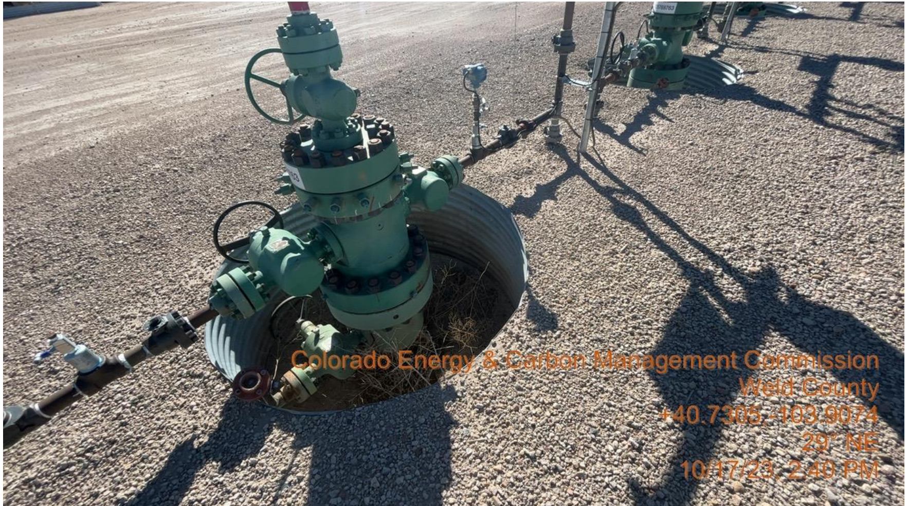
Photo 7. The photo was taken on the well location facing Northeast. The photo illustrates uncovered cellars around the wellheads.
