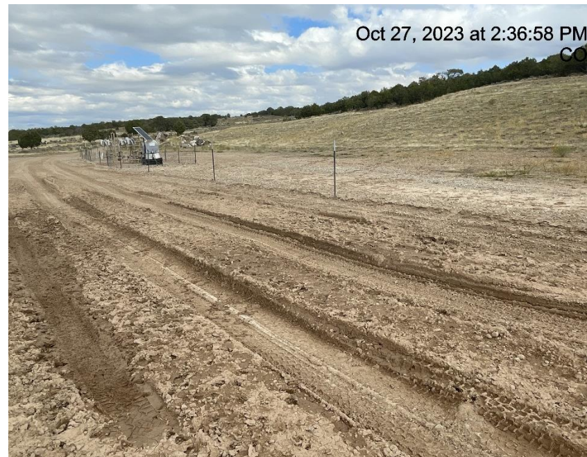
Photo # 4721 Lack of stabilization/compaction/insufficient BMP's
