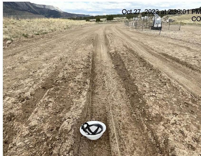
Photo # 4713 Lack of stabilization/compaction/insufficient BMP's
