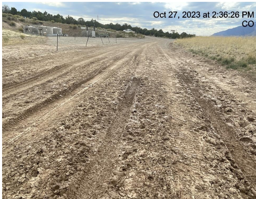
Photo # 4716 Lack of stabilization/compaction/insufficient BMP's
