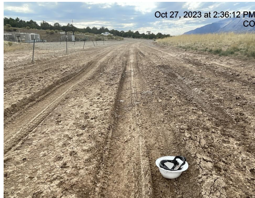
Photo # 4715 Lack of stabilization/compaction/insufficient BMP's
