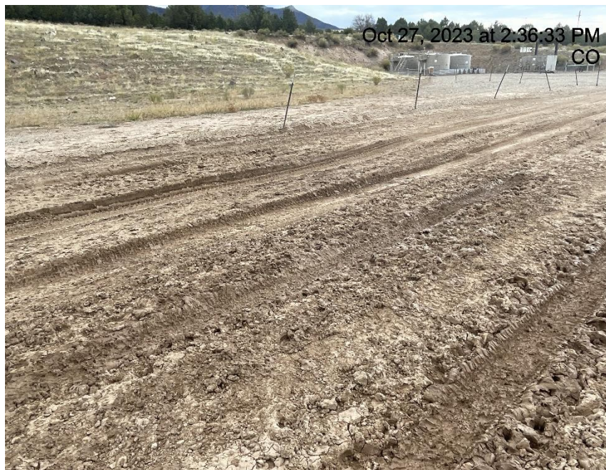
Photo # 4718 Lack of stabilization/compaction/insufficient BMP's
