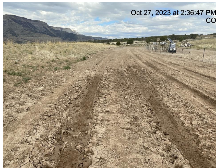
Photo # 4719 Lack of stabilization/compaction/insufficient BMP's
