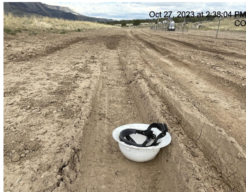
Photo # 4723 Lack of stabilization/compaction/insufficient BMP's
