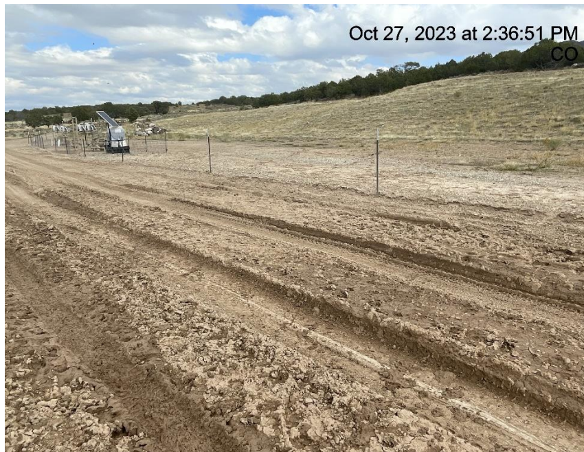
Photo # 4720 Lack of stabilization/compaction/insufficient BMP's
