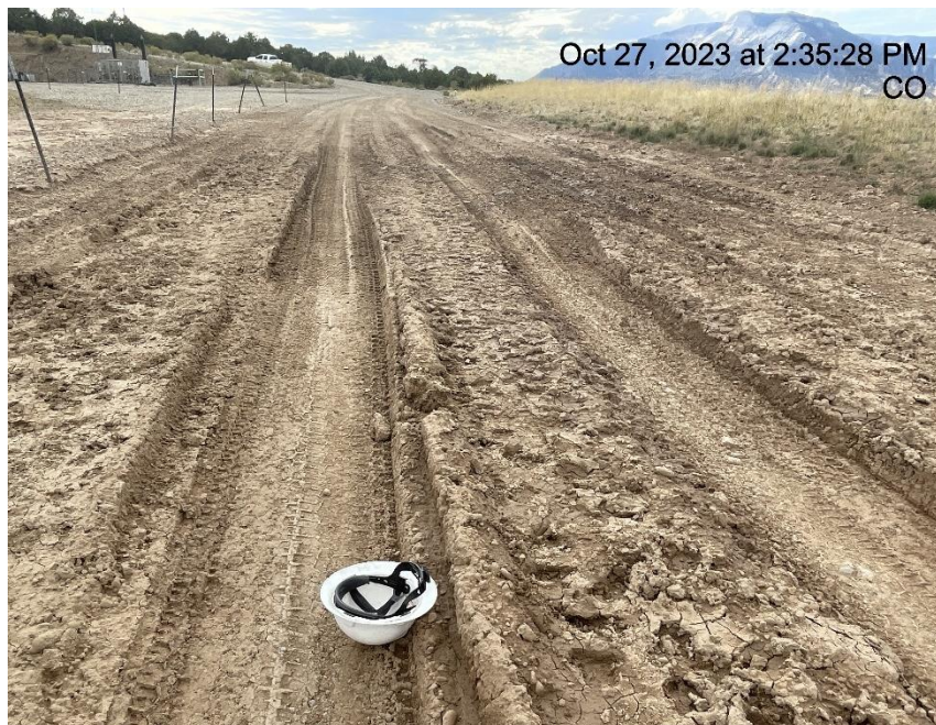
Photo # 4710 Lack of stabilization/compaction/insufficient BMP's
