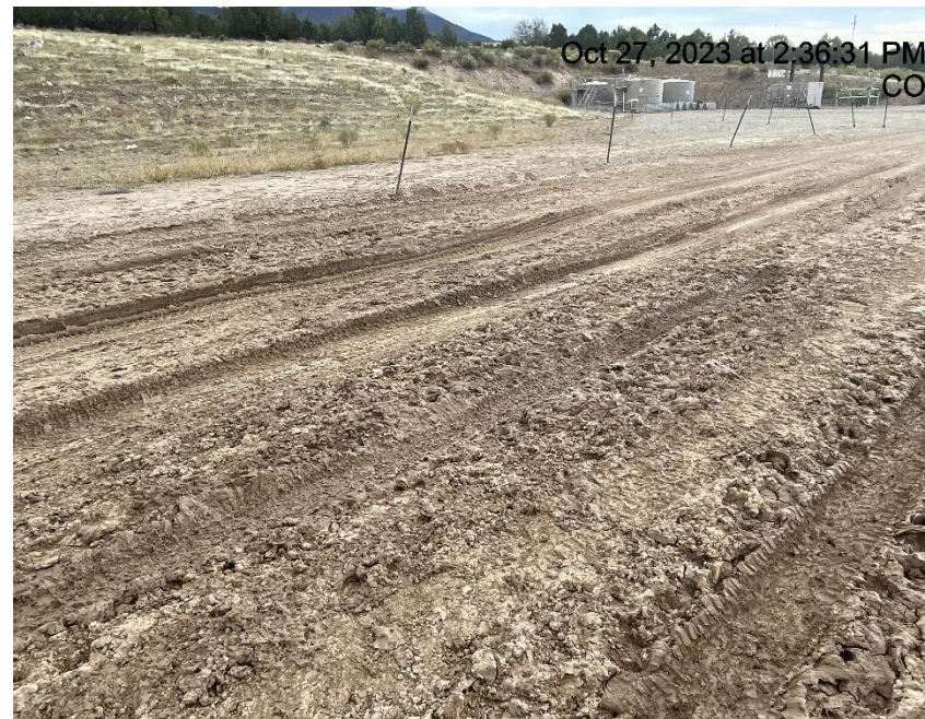
Photo # 4717 Lack of stabilization/compaction/insufficient BMP's
