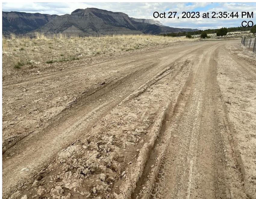
Photo # 4712 Lack of stabilization/compaction/insufficient BMP's
