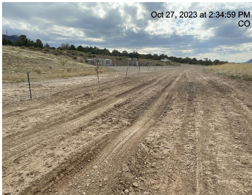
Photo # 4706 Lack of stabilization/compaction/insufficient BMP's
