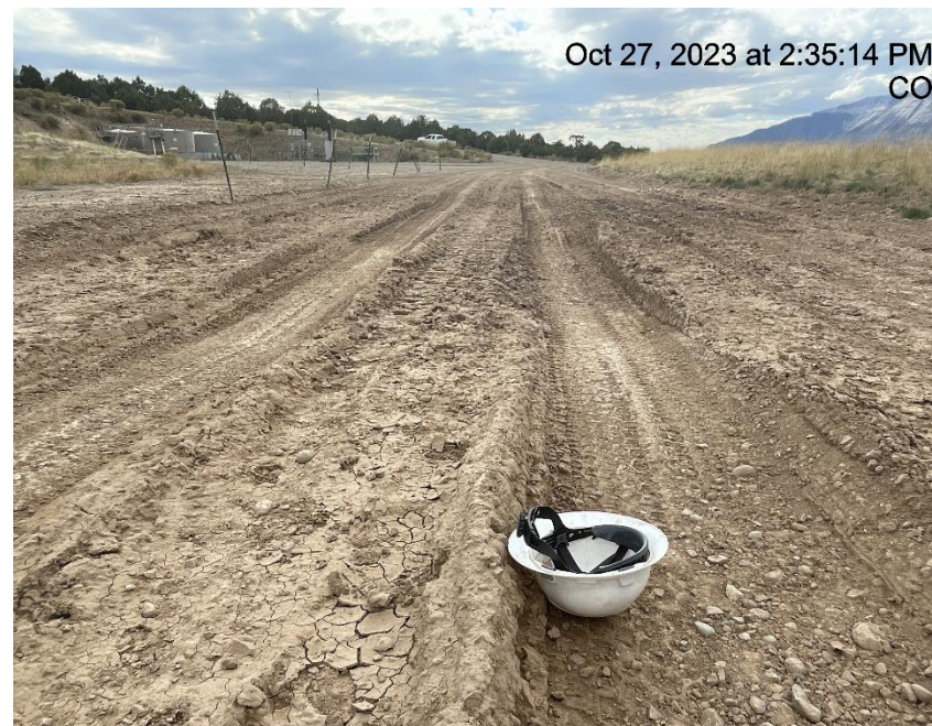
Photo # 4709 Lack of stabilization/compaction/insufficient BMP's
