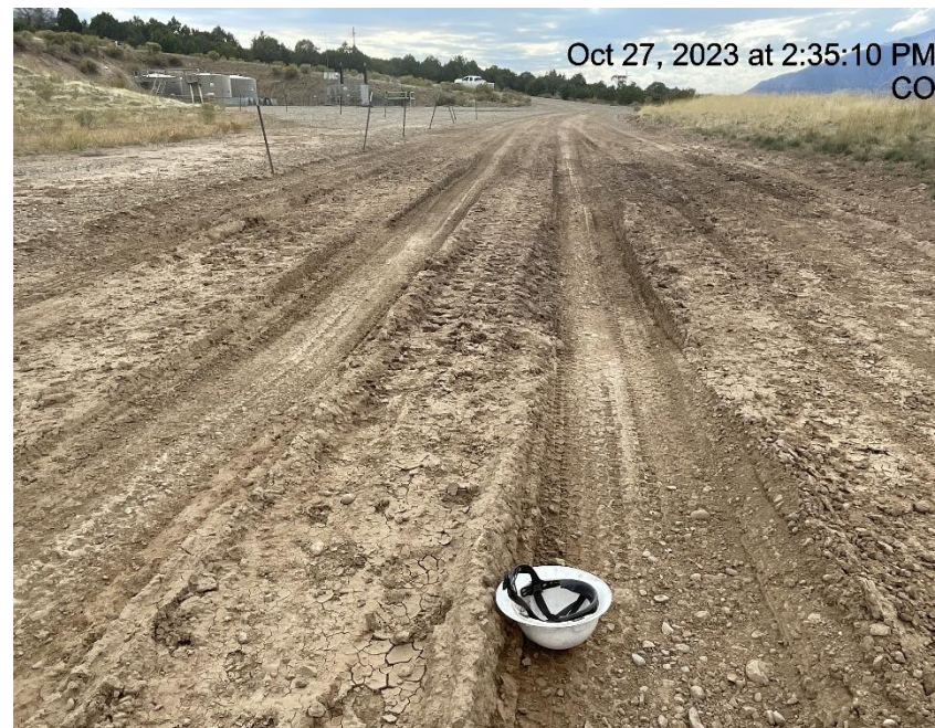
Photo # 4707 Lack of stabilization/compaction/insufficient BMP's
