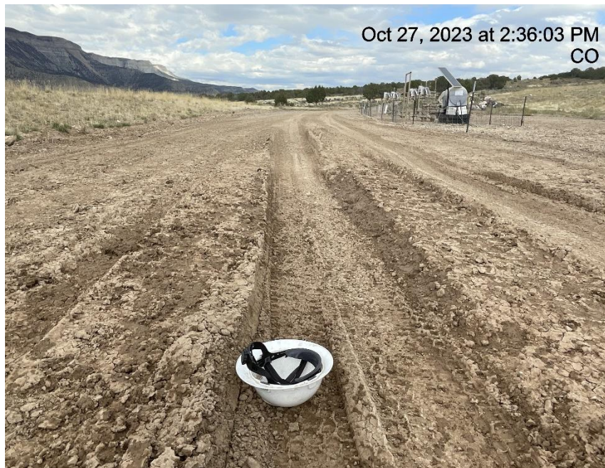
Photo # 4714 Lack of stabilization/compaction/insufficient BMP's
