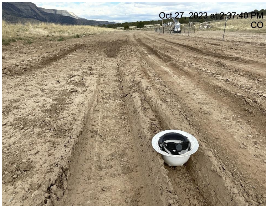
Photo # 4722 Lack of stabilization/compaction/insufficient BMP's
