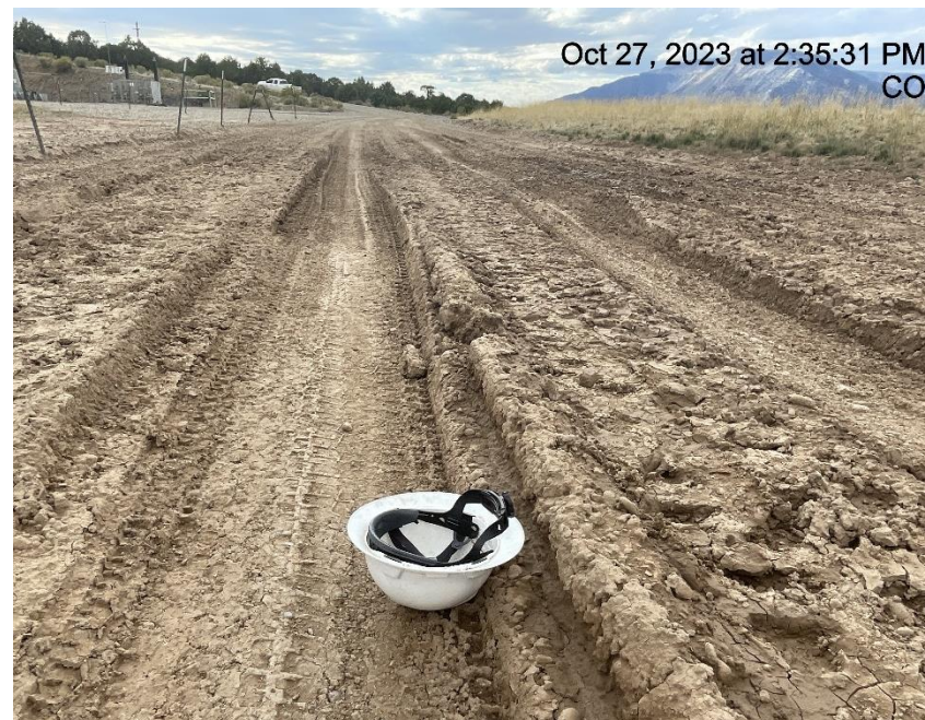
Photo # 4711 Lack of stabilization/compaction/insufficient BMP's
