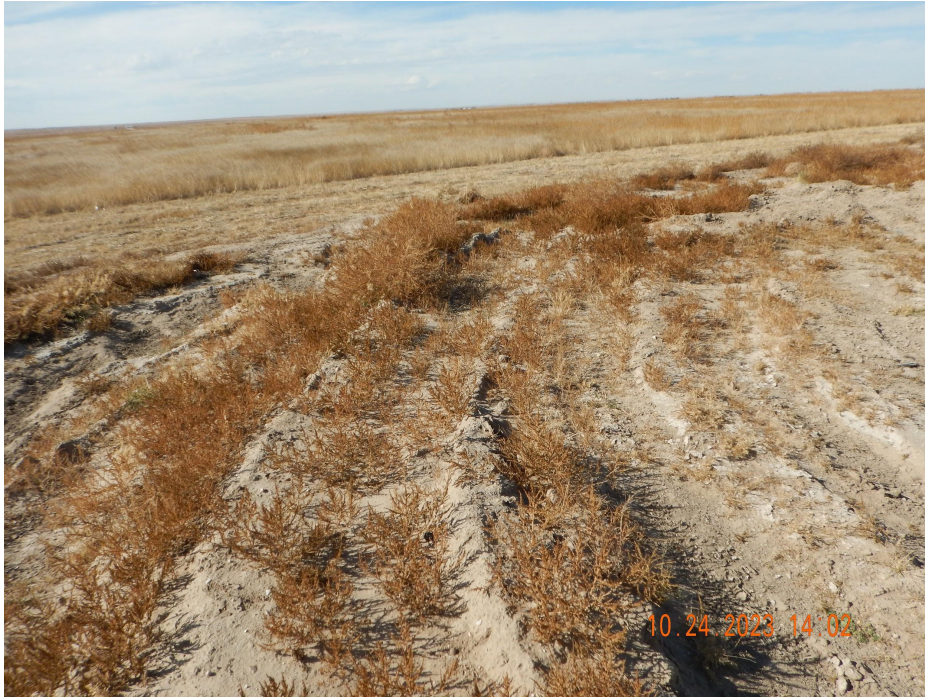
Photo 7. Photo taken from the southwestern location facing West. Photo illustrates that there was not a sufficient response to install stormwater BMPs to prevent sediment laden stormwater from discharging off location. The ditch and berm by itself is not sufficient and it has not been constructed with good engineering practices.
