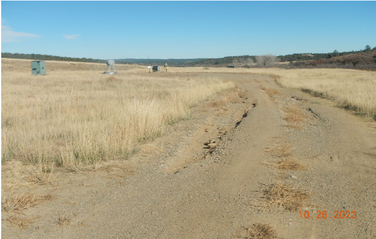
Photo 1. Facing east toward the access road. There is erosion that needs to be repaired.
