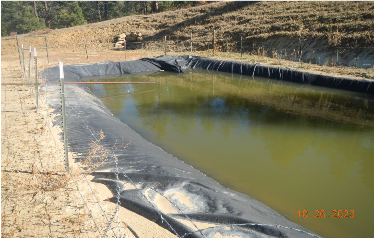
Photo 3. Facing toward the pit. No freeboard marker present..
