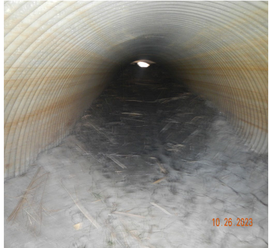
Photo 2. The two culvert crossing the drainage remain filled in with sediment.
