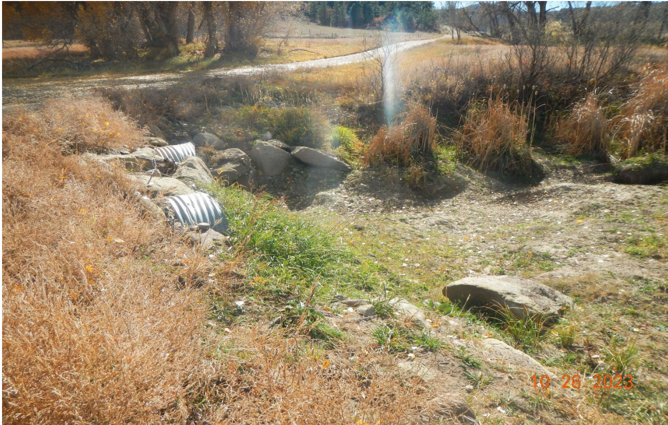
Photo 1. The two culvert crossing the drainage remain filled in with sediment.
