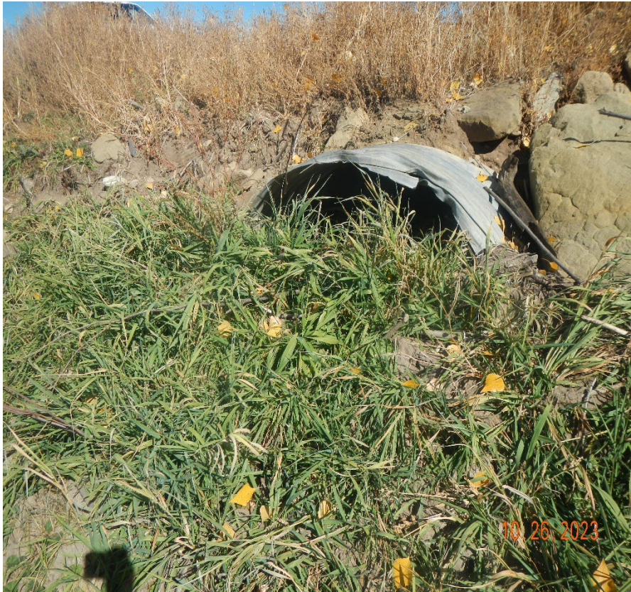
Photo 2. The two culvert crossing the drainage remain filled in with sediment.
