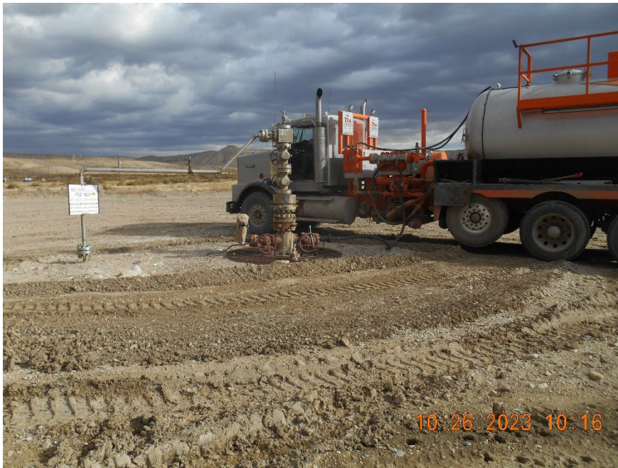
Injection well during MIT
