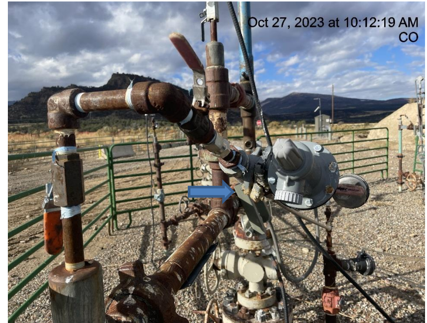
Photo # 4419 Bracket on little joe regulator broken
