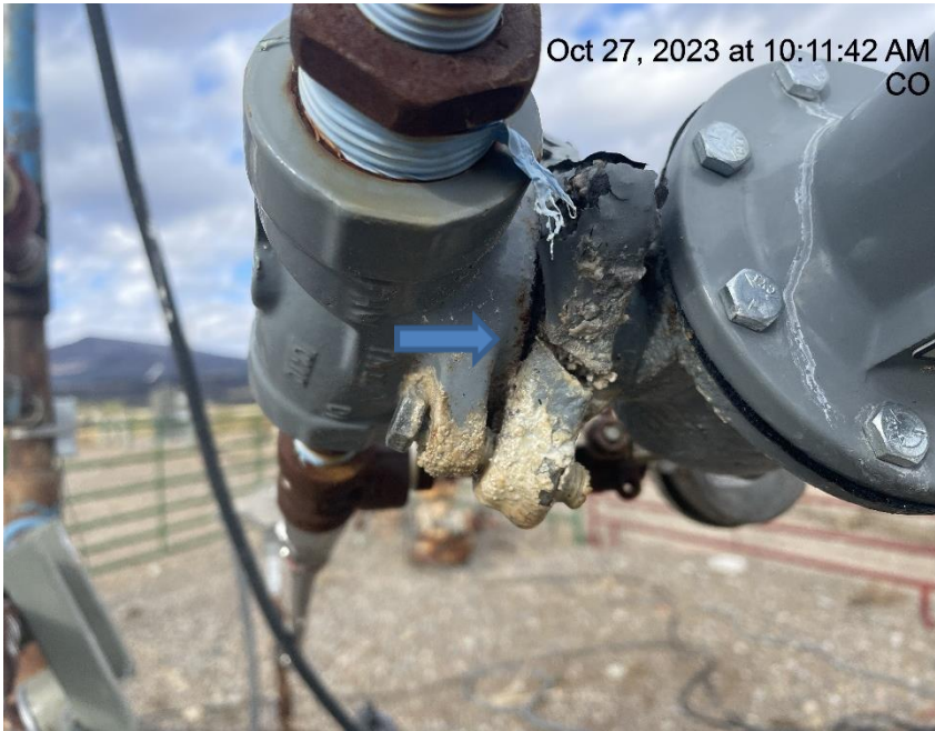
Photo # 4420 Bracket on little joe regulator broken
