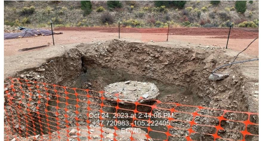
**Photo 3 – SMU 4-4-P Cemented Wellhead,
