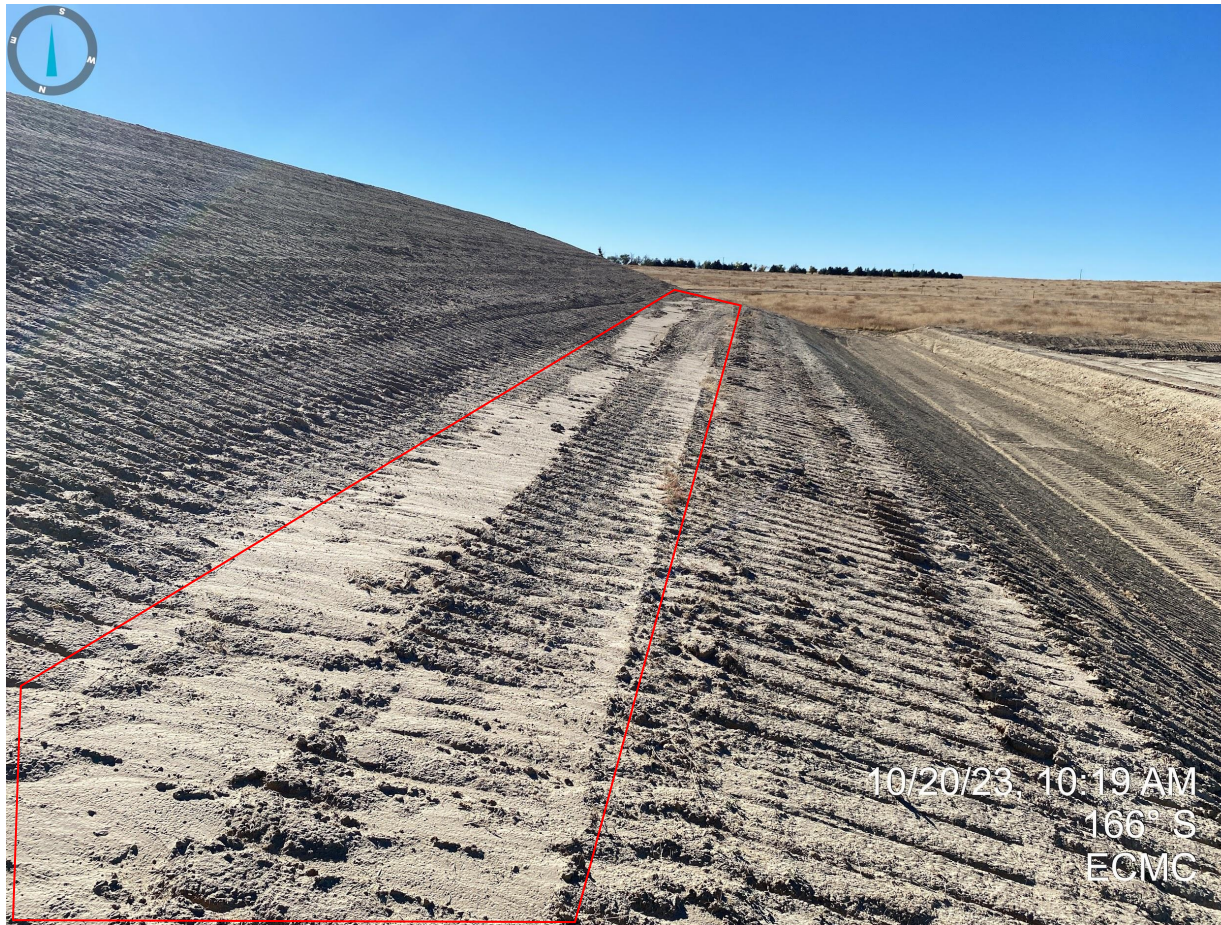
Photo 26. Taken from the east side of the topsoil stockpile. Photo illustrates evidence of sediment transport/deposition from improper temporary tracking and no apparent stormwater controls/BMPs to prevent topsoil from migrating into the adjacent stormwater ditch. Additional perimeter controls are required to prevent erosion degradation.
