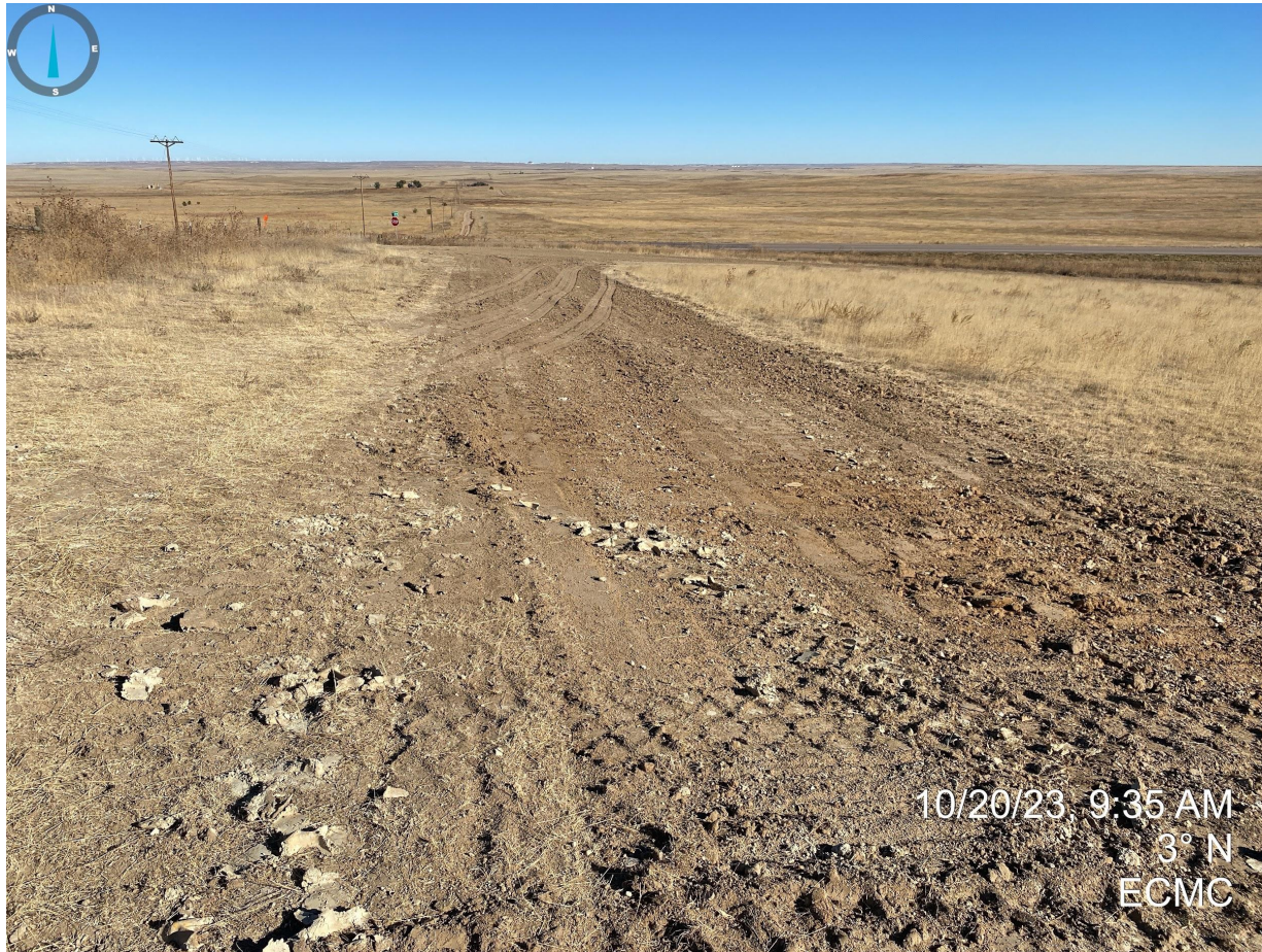
Photo 5. Taken north of the new entrance/access road. Photo illustrates a portion of the former access road that has had topsoil added for subsequent reclamation. Onsite Operator representative informed Staff that topsoil salvaged from the new access road was redistributed throughout the former access road. Soils pictured here are not properly stabilized against wind/water erosion degradation.
