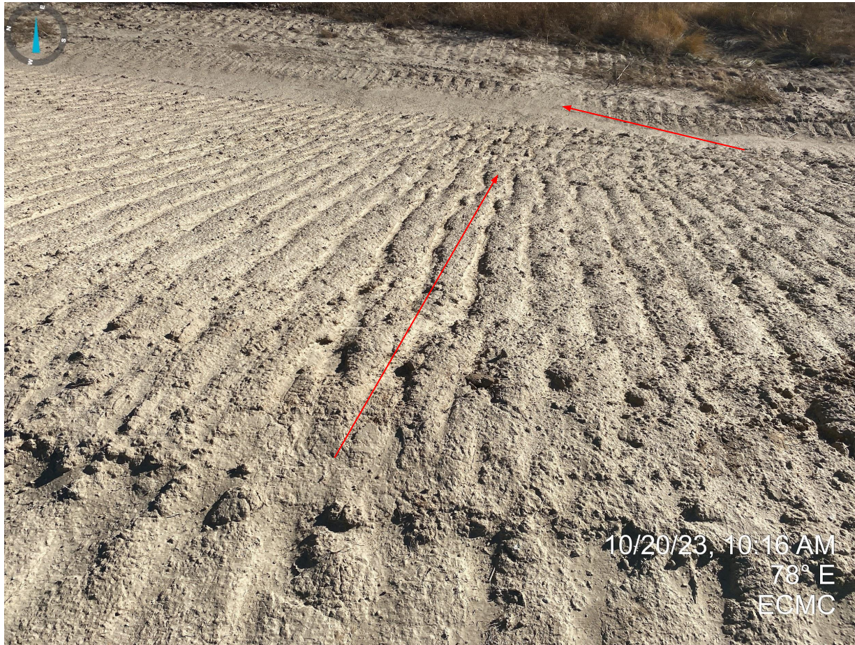
Photo 25. Erosion degradation (e.g. rilling) observed on the east side of the topsoil stockpile. Evidence of sediment deposition and absence of perimeter stormwater controls around the stockpile.
