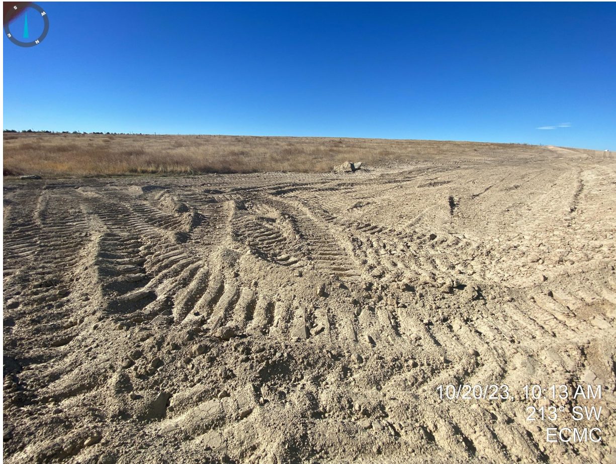
Photo 21. Unstabilized soils observed southeast of the production pad.
