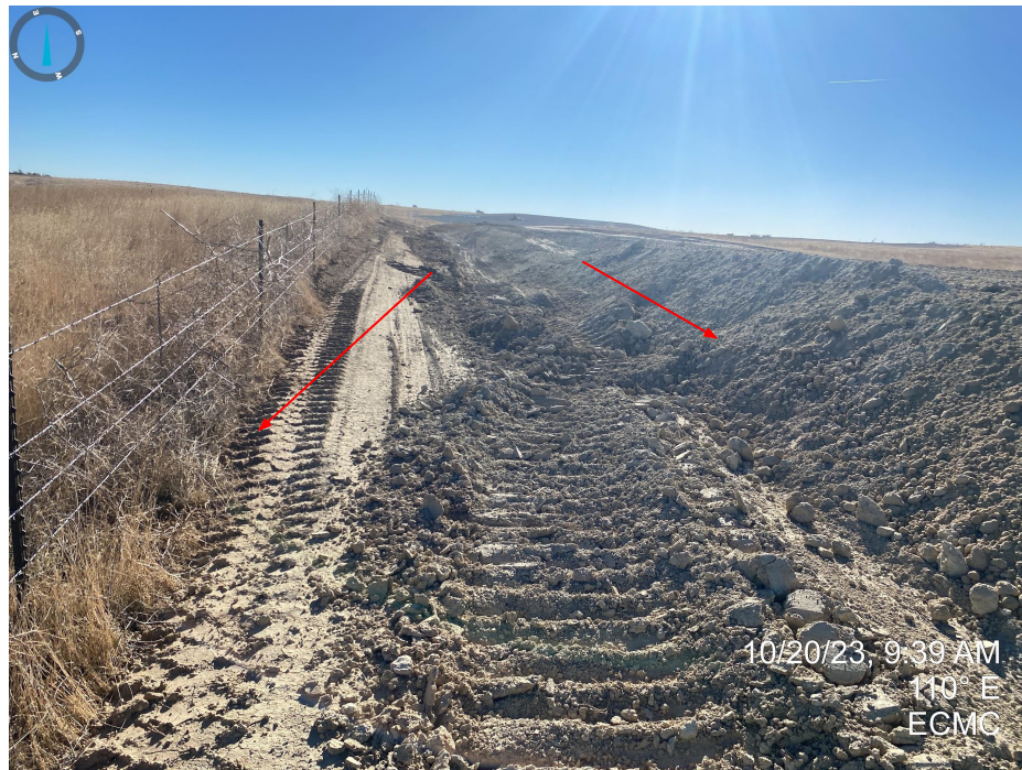
Photos 12 & 13. Continued from Photos 10 & 11. Unconsolidated material and the absence of perimeter stormwater control measures/BMPs.
