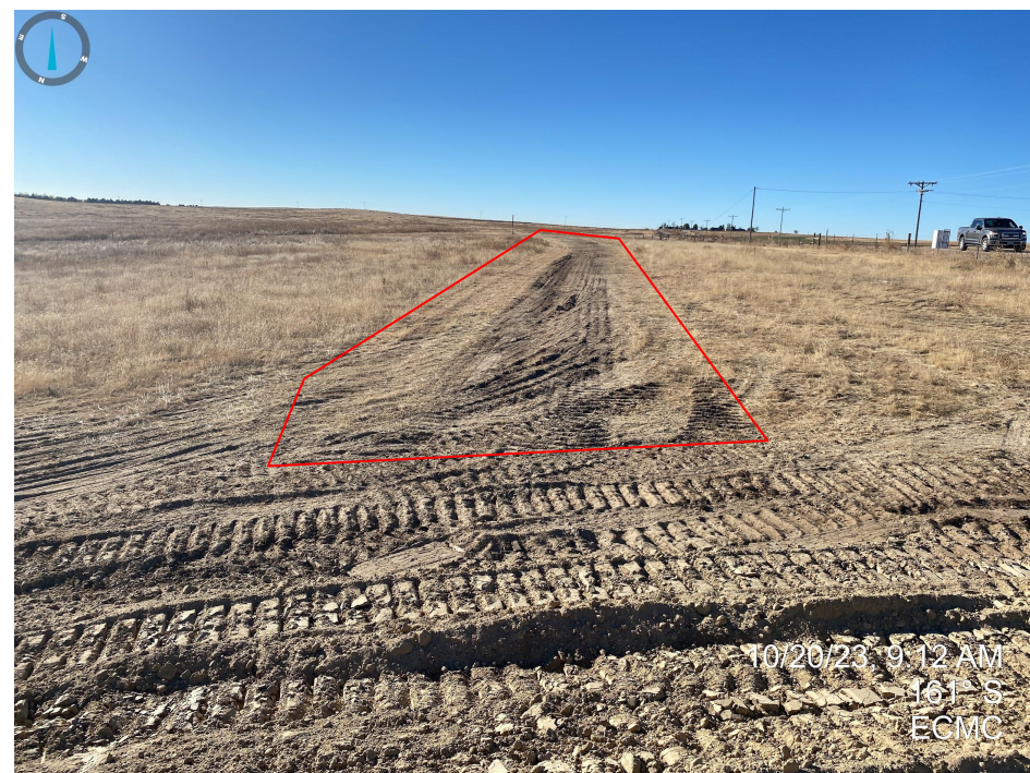
Photos 1 & 2. Previously used access roads, south of the new access road, have been disturbed by vehicle and construction activities. These disturbances will need to be reclaimed per the 1000 series rules.
