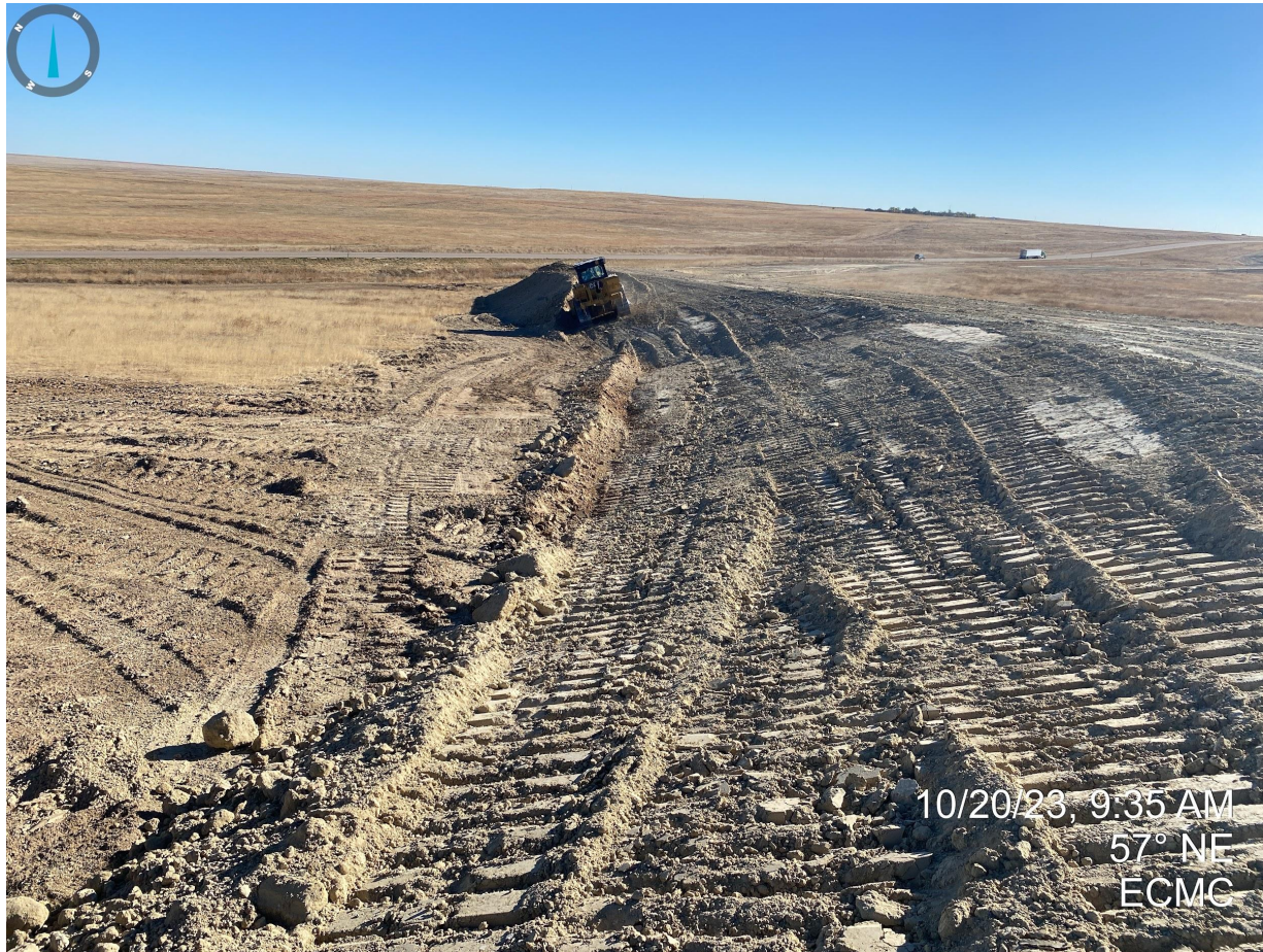
Photo 4. Taken from the new location entrance. Photo illustrates fine grading of the new access road. Also pictured, equipment tracking is parallel to the slope. Additional stabilization techniques (e.g. seeding/mulching) should be implemented to protect the soils from wind and water erosion degradation. .
