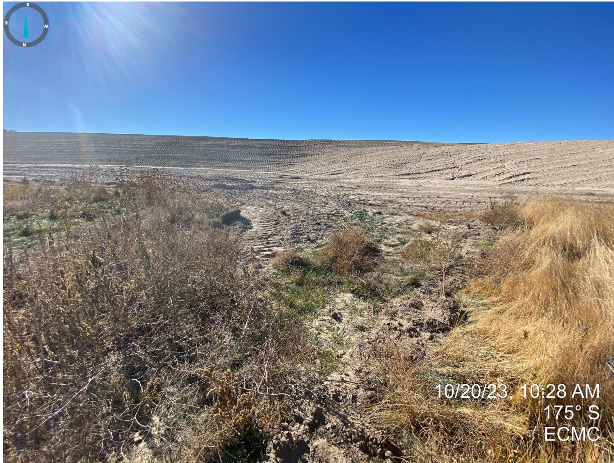
Photo 30. Erosion degradation previously documented does not appear to have been repaired, and no additional stormwater control measures observed that would prevent/manage stormwater from exiting off location into adjacent areas. Additional and more robust control measures are required as much of the stormwater from the location could potentially collect in this low spot.
