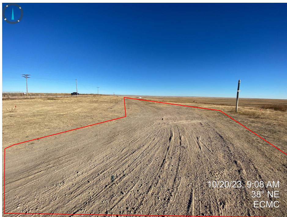
Photos 1 & 2. Previously used access roads, south of the new access road, have been disturbed by vehicle and construction activities. These disturbances will need to be reclaimed per the 1000 series rules.
