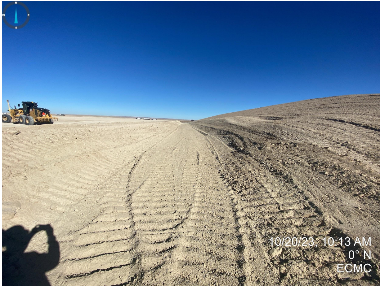
Photo 20. Taken from the southeastern portion of the production pad. Photo illustrates the absence of stormwater controls/BMPs within the stormwater ditch that would help to reduce the velocity of stormwater.
