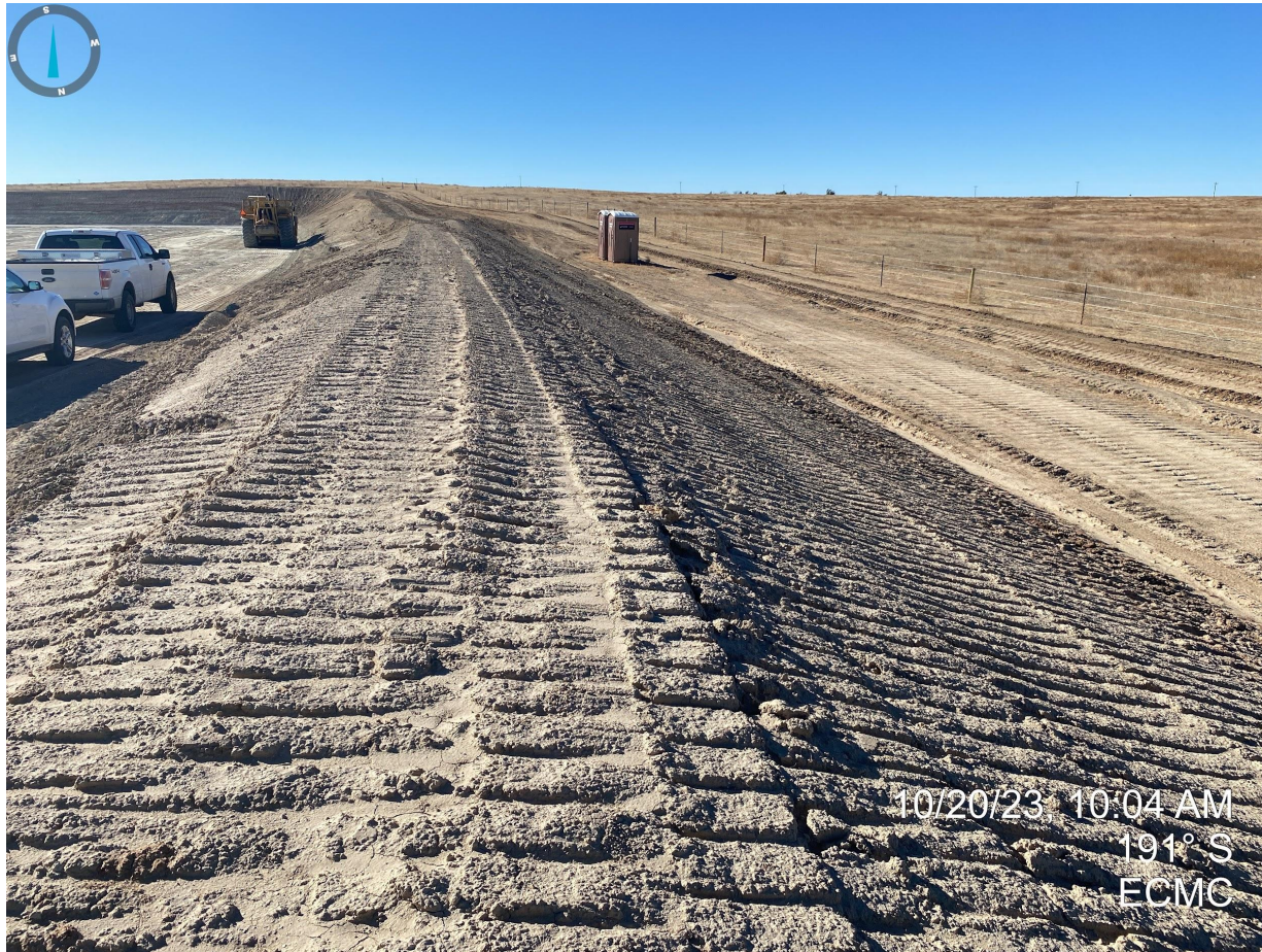
Photo 16. Taken from the northwest corner of the location. Photo illustrates that equipment tracking is parallel to the slope.
