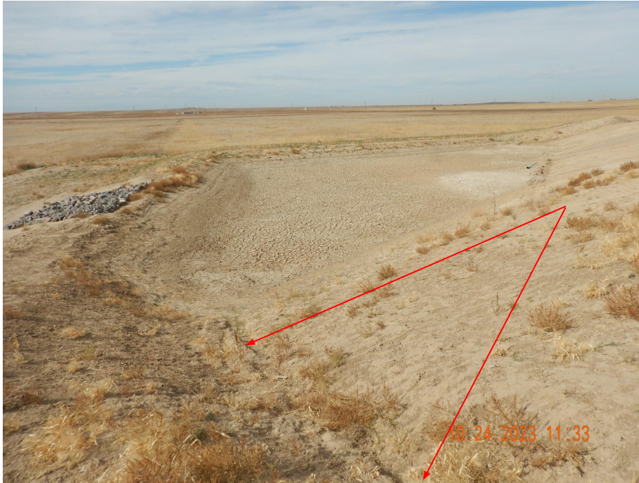
Photo 9. Photo taken from the southwestern portion of the location, facing West. Photo illustrates a detention area that is in proper functioning condition.
