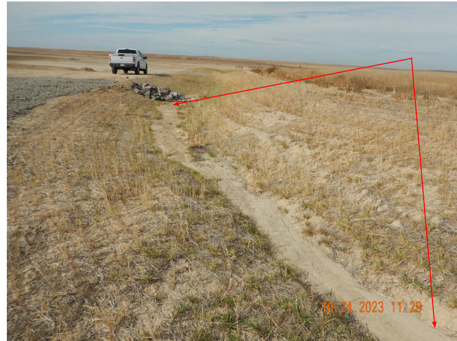
Photo 4. Photo taken from Photo 3, facing West. Photo illustrates sediment accumulation in the roadside ditch areas.
