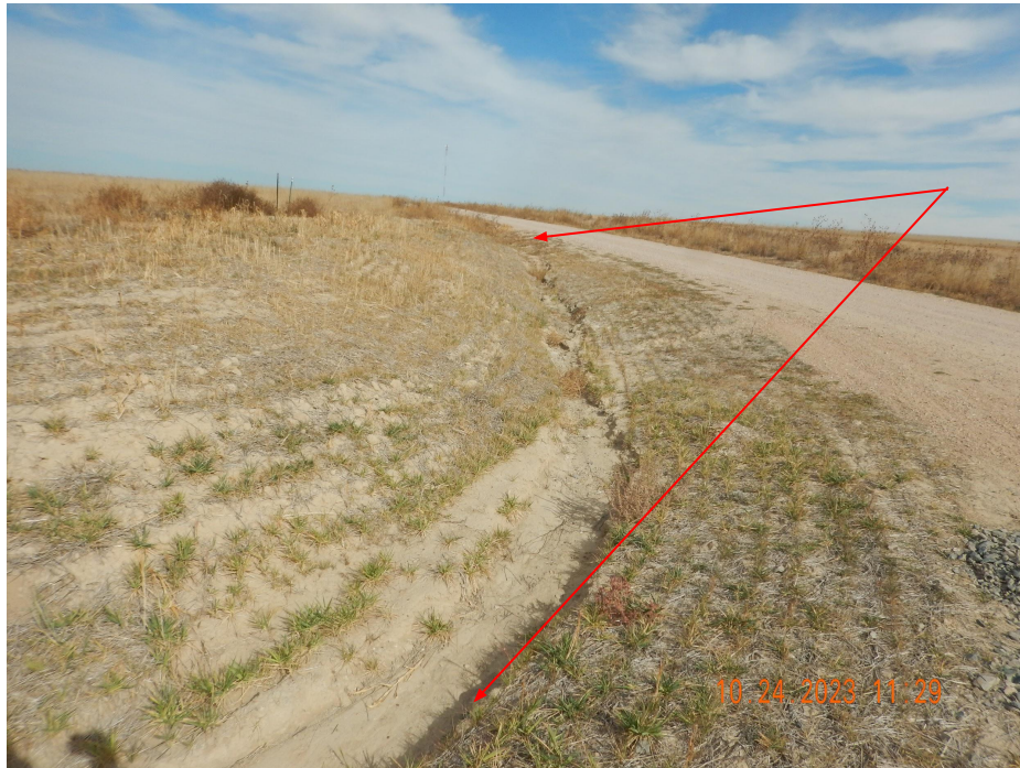
Photo 3. Photo taken from the entrance of location, facing North. Photo illustrates stormwater erosion which needs additional BMPs and repairs.
