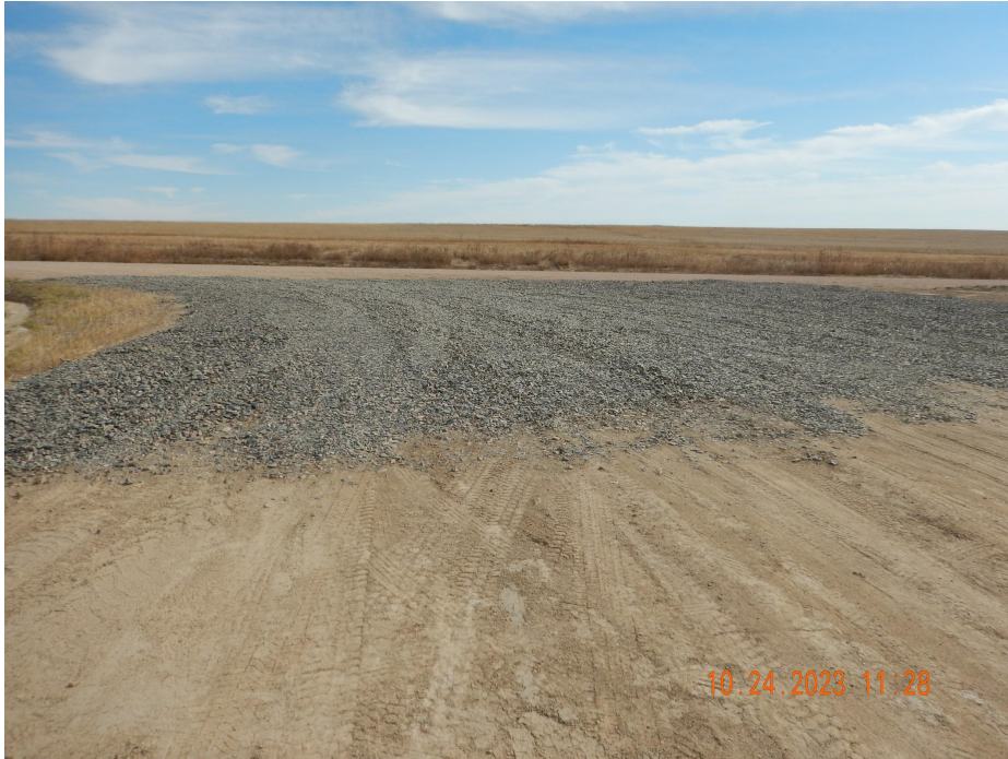
Photo 1. Photo taken from the entrance of location, facing East. Photo illustrates a tracking device BMP installed. At the time of this inspection, the BMP was in proper functioning condition.
