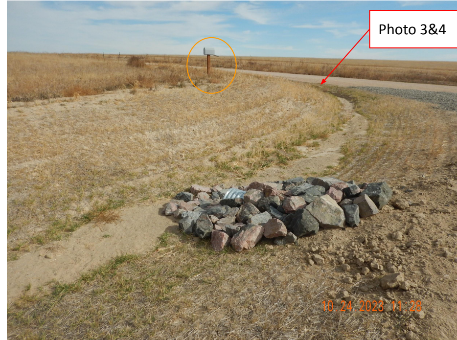
Photo 2. Photo taken from the entrance of location, facing Northeast. Photo illustrates inlet culvert protection. However, there was erosion observed along the roadside ditch area.
