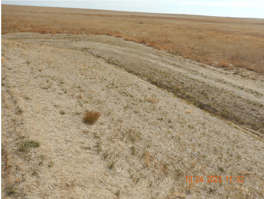
Photo 7. Photo taken from the southeastern location on the topsoil stockpile, facing Southeast. Photo illustrates Operator has installed a perimeter ditch BMP in response to the previous corrective action.
