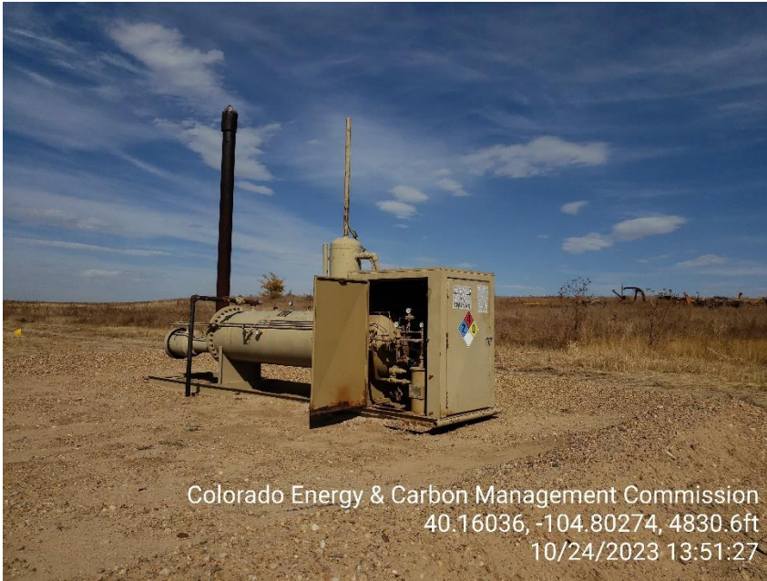
Photo 9 Horizontal Heated Separator.
