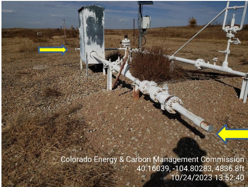
Photo 11 Unused Gas Meter Run.
