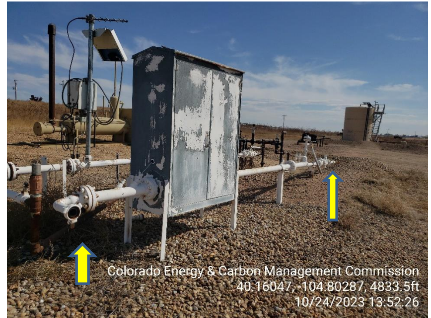
Photo 12 Unused Gas Meter Run.
