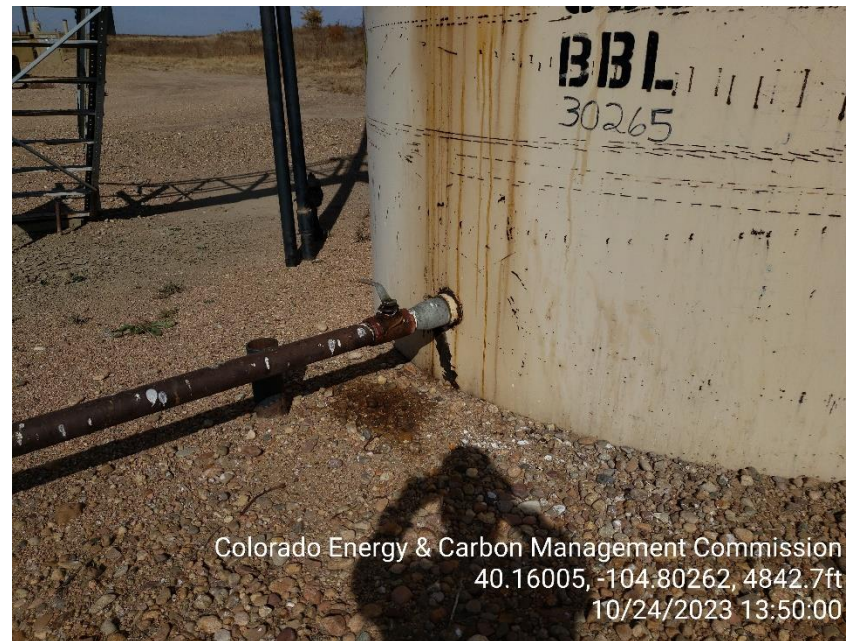
Photo 4 Stained soil by load out valve.
