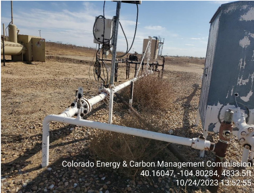
Photo 13 Gas Meter Run.
