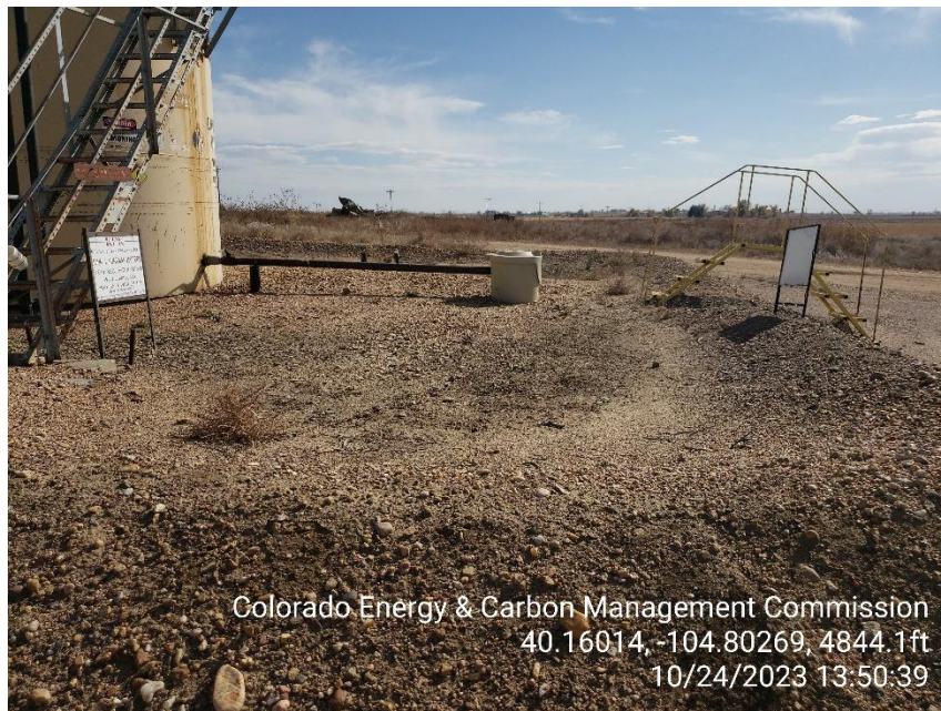
Photo 7 TB inside berm is near level.
