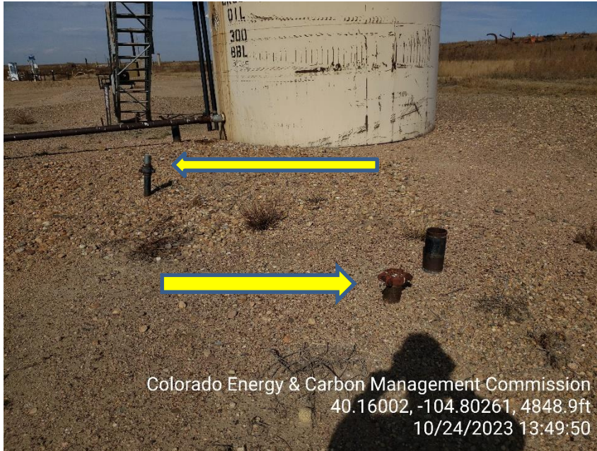
Photo 5 Unmarked flow lines.
