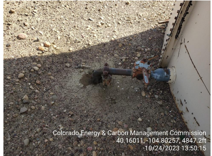
Photo 6 Stained soil by crude oil valve back side.
