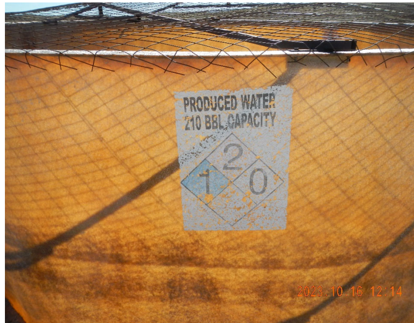
6. Faded Content/Quantity/Hazard label on produced water tank.
