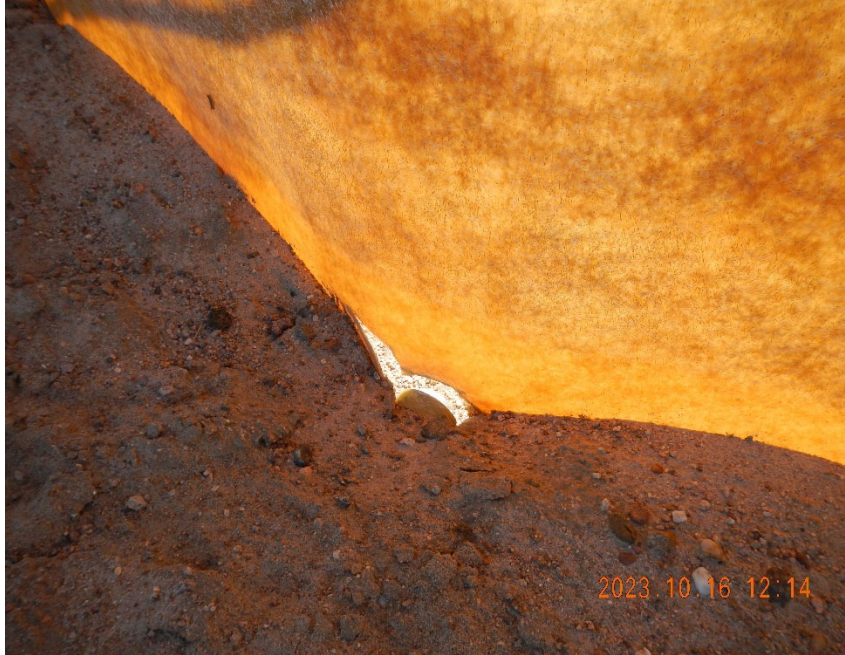
7. Hole in the produced water tank wall.
