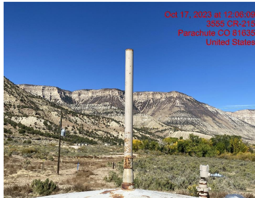
Open-Ended Tank Vent – Photo #07033
