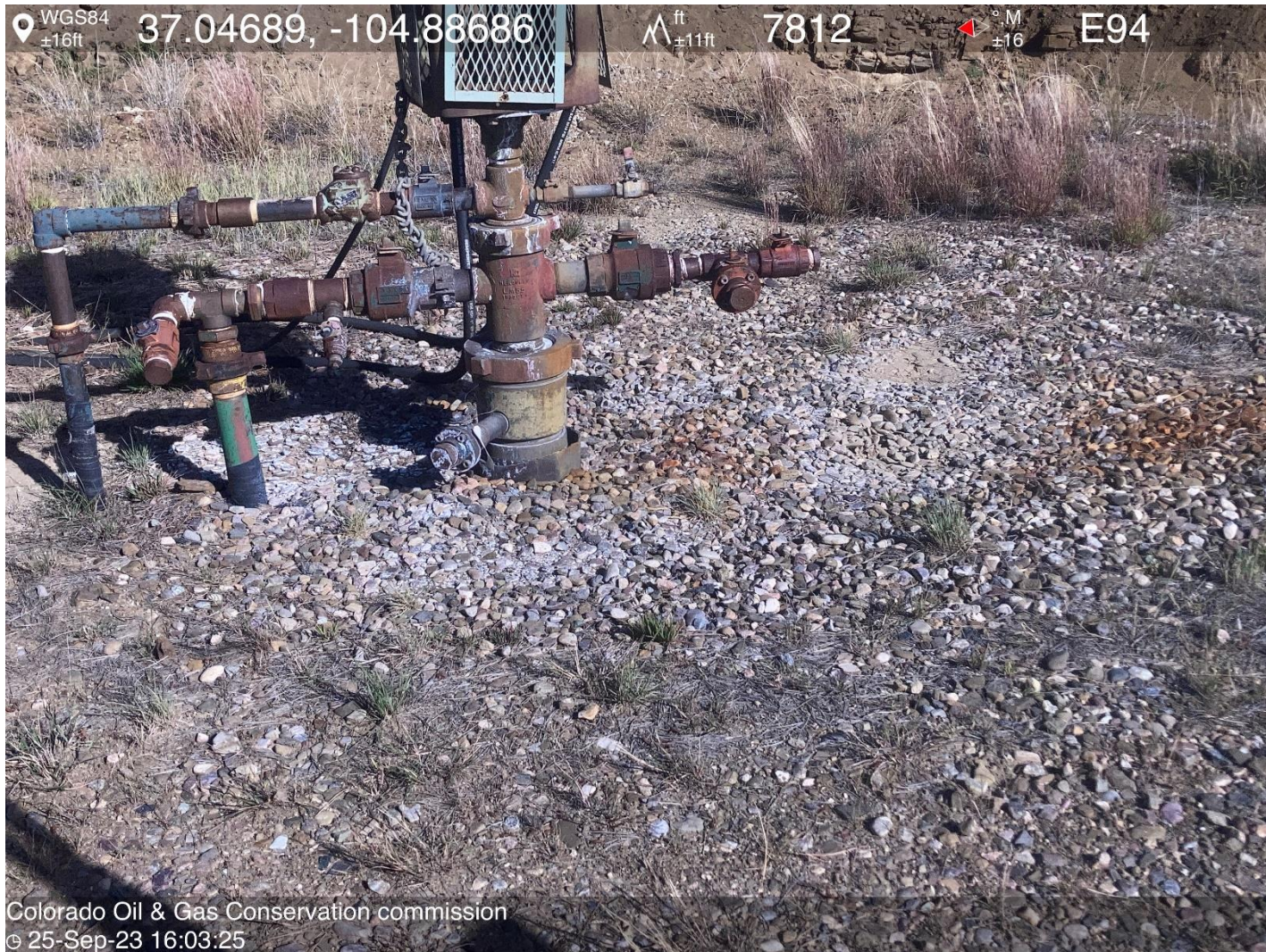
PHOTO 4: Produced water spill from the wellhead has left a salt impacted area around the wellhead. Securely fasten all valves, pipes, fittings, and Production Facilities to ensure good mechanical condition, inspect at regular intervals and maintain in good mechanical condition remove and dispose of impacted material per Rule 608.e. CA DATE 11-20-2023.
