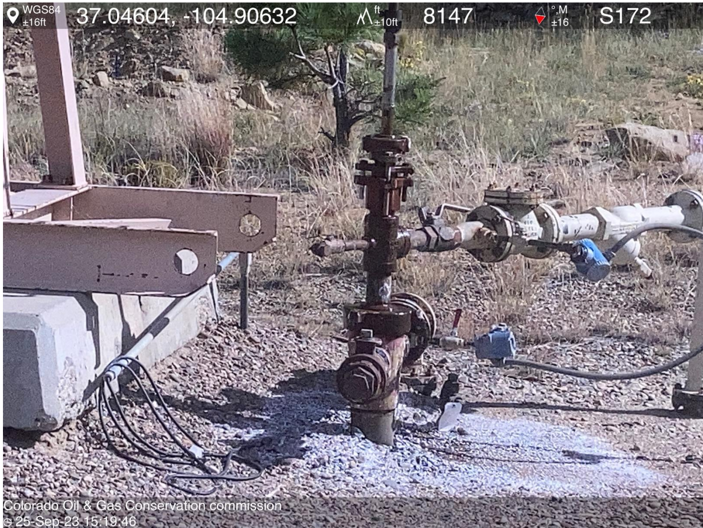
PHOTO 5: Signs of recent slow leak from wellhead. Salt/mineral buildup is evident on the wellhead ground around wellhead. Securely fasten all valves, pipes, fittings, and Production Facilities to ensure good mechanical condition, inspect at regular intervals, remove salt/mineral buildup, remove and dispose of impacted material and maintain in good mechanical condition per Rule 608.e. ca date 11-20-2023.
