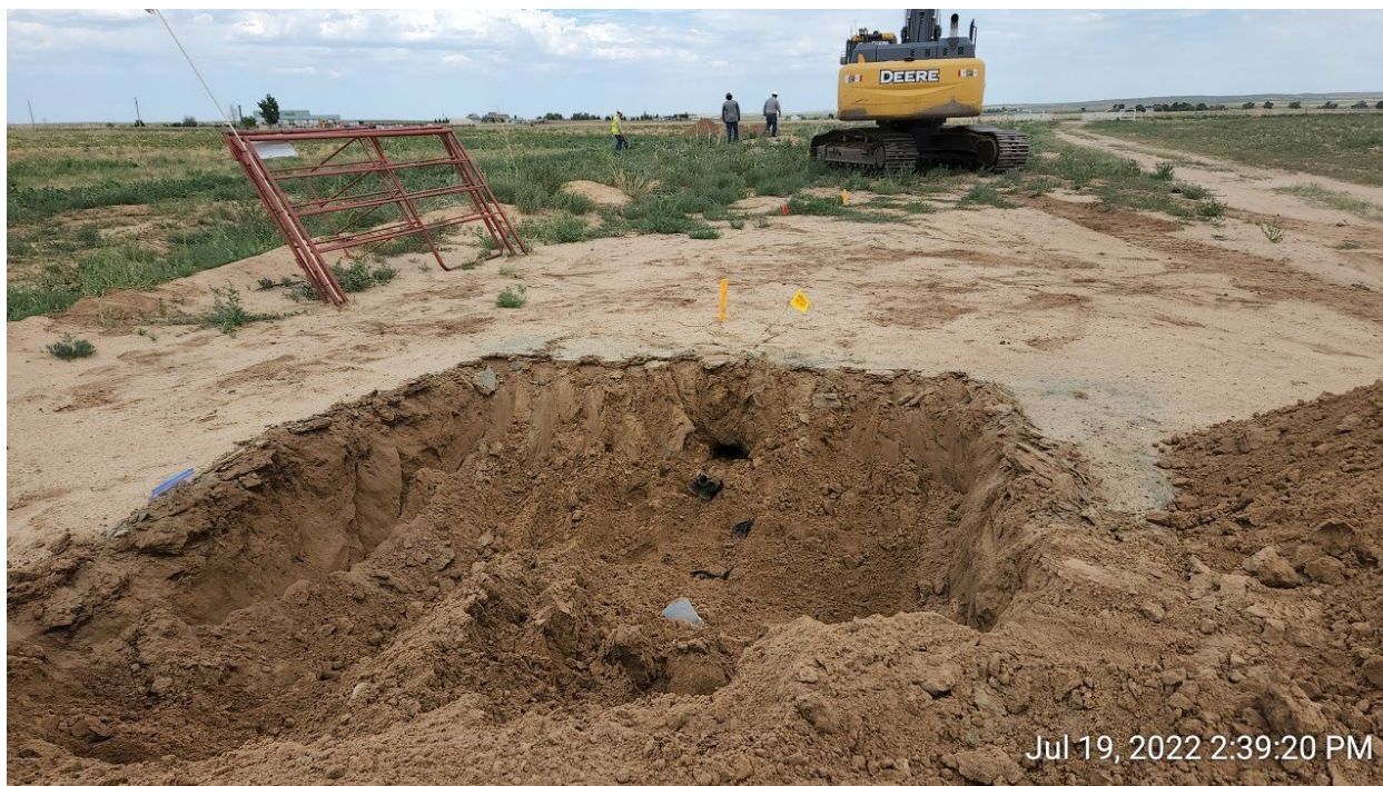
#1A – PTF C 32-8 Flowline Removal – 8FL01@3.0' – Wellhead Tie-in - No Impacts Noted - PID 0.3ppm
