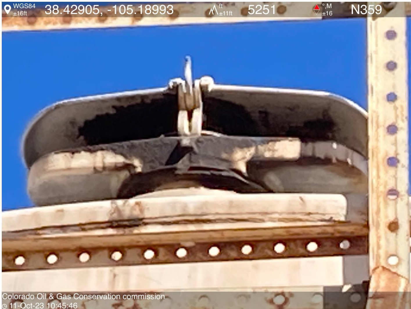
PHOTO 9: GAUGE HATCH OPEN OR NOT SEALED ON BOTH CRUDE OIL TANKS. Close and seal gauge hatches when not accessing tank per Rule 608.a.(9). THIS IS THE SECOND NOTICE FOR THIS CORRECTIVE ACTION IMMEDIATE ACTION IS REQUIRED.
