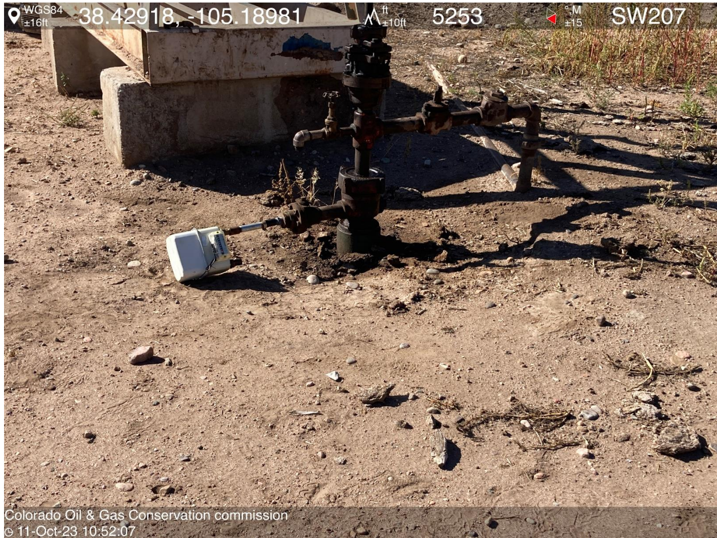
PHOTO 11: Bradenhead inaccessible or not visible. Install appropriate fittings to allow bradenhead visual inspection as per Rule 419.a.(1), (2). THIS IS THE SECOND NOTICE FOR THIS CORRECTIVE ACTION, IMMEDIATE ACTION IS REQUIRED.
