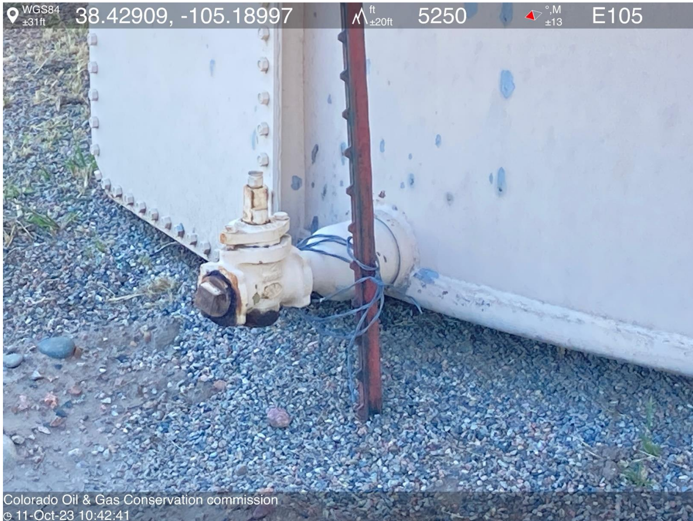
PHOTO 13: Equipment in geologic hazard area not anchored or inadequately anchored. Anchor equipment ensuring anchors are (engineered) to ensure the equipment will resist flotation, collapse, lateral movement, or subsidence per Rule 607. THIS IS THE SECOND NOTICE FOR THIS CORRECTIVE ACTION, IMMEDIATE ACTION IS REQUIRED. NOTE: PER RULE ANCHORING MUST BE ENGINEERED.
