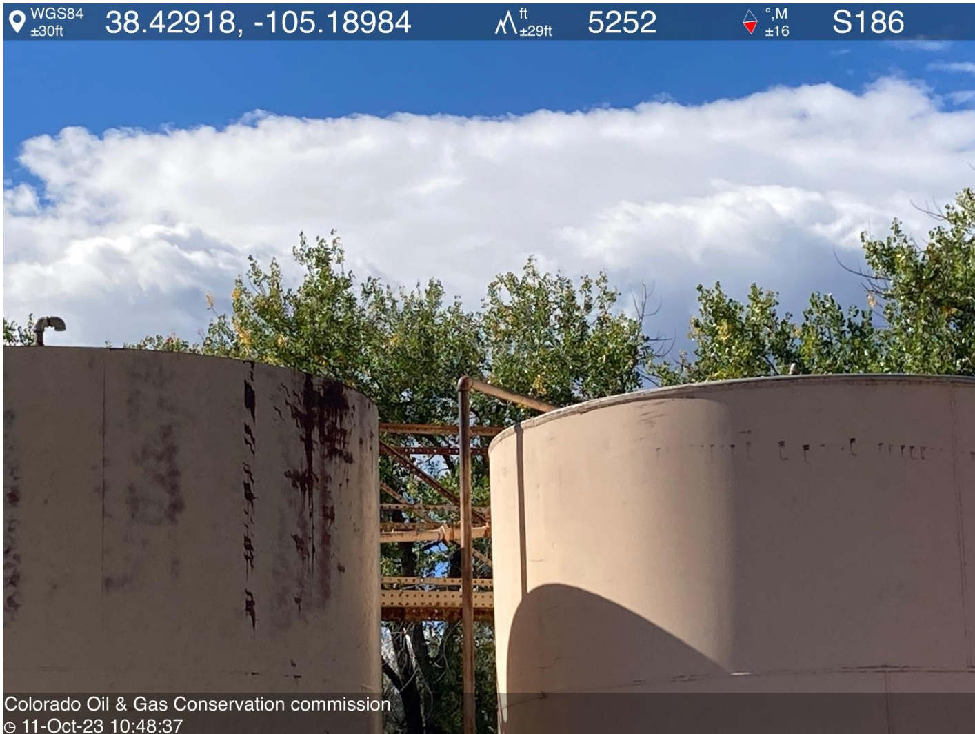
PHOTO 8: THERE IS A 2" PIPE ON THE JJ#2 TANK BATTERY OPENENDED AND NO PRESSURE RELIEF VALVE INSTALLED. Tanks will function as sealed and ventless with gas released only through a vapor control system or properly sized pressure relief valve. per Rule 608.a.(9). CA DATE 11-11-2023.
