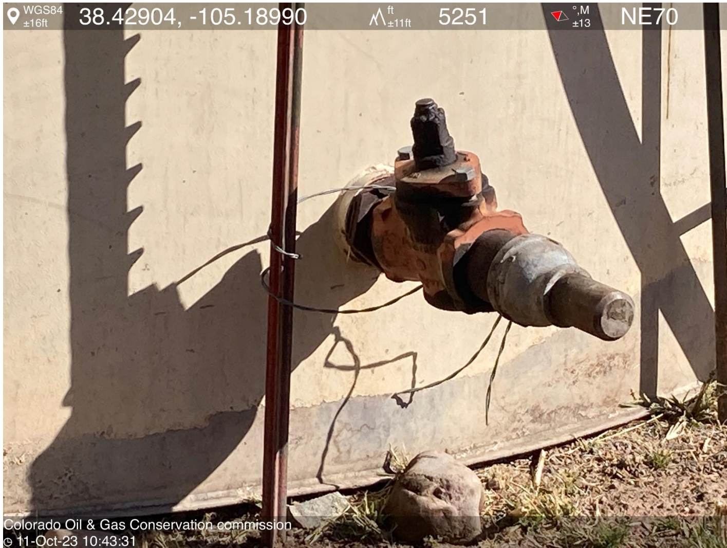
PHOTO 12: Equipment in geologic hazard area not anchored or inadequately anchored. Anchor equipment ensuring anchors are (engineered) to ensure the equipment will resist flotation, collapse, lateral movement, or subsidence per Rule 607. THIS IS THE SECOND NOTICE FOR THIS CORRECTIVE ACTION, IMMEDIATE ACTION IS REQUIRED. NOTE: PER RULE ANCHORING MUST BE ENGINEERED.
