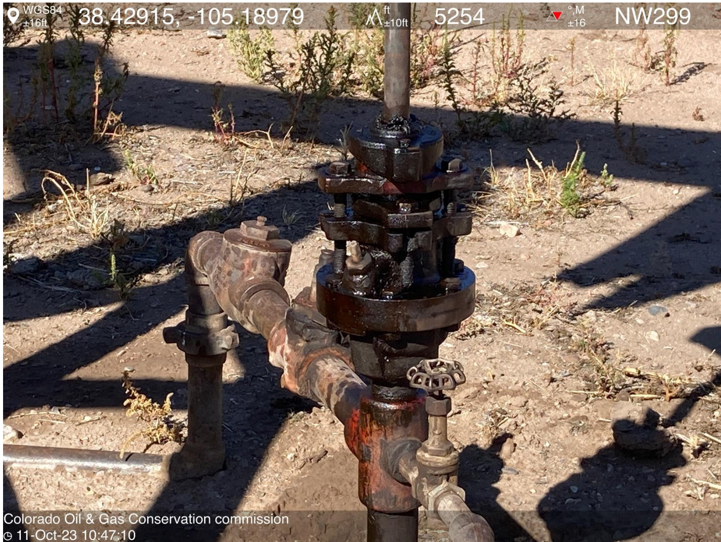
PHOTO 7: POLISH ROD PACKING LEAK. Securely fasten all valves, pipes, fittings, and Production Facilities to ensure good mechanical condition, inspect at regular intervals and maintain in good mechanical condition per Rule 608.e. Securely fasten all valves, pipes, fittings, and Production Facilities to ensure good mechanical condition, inspect at regular intervals and maintain in good mechanical condition per Rule 608.e. CA DATE 11-11-2023.
