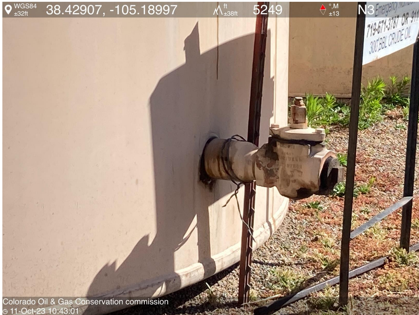
PHOTO 14: Equipment in geologic hazard area not anchored or inadequately anchored. Anchor equipment ensuring anchors are (engineered) to ensure the equipment will resist flotation, collapse, lateral movement, or subsidence per Rule 607. THIS IS THE SECOND NOTICE FOR THIS CORRECTIVE ACTION, IMMEDIATE ACTION IS REQUIRED. NOTE: PER RULE ANCHORING MUST BE ENGINEERED.
