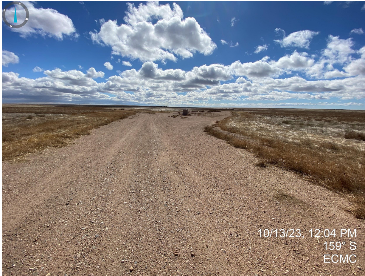
Photo 1. Taken near the entrance. It does not appear any reclamation work has been conducted. Access road/road base material remains on location.
