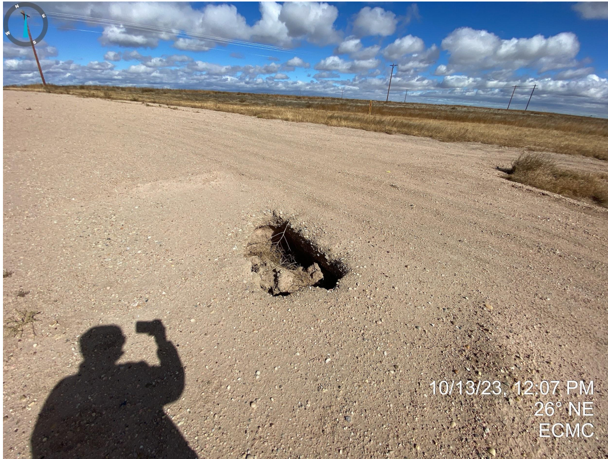
Photo 3. Subsidence/hole was observed on the former production facilities. The Operator was immediately contacted and instructed to mark/cover the opening to ensure safe operations.
