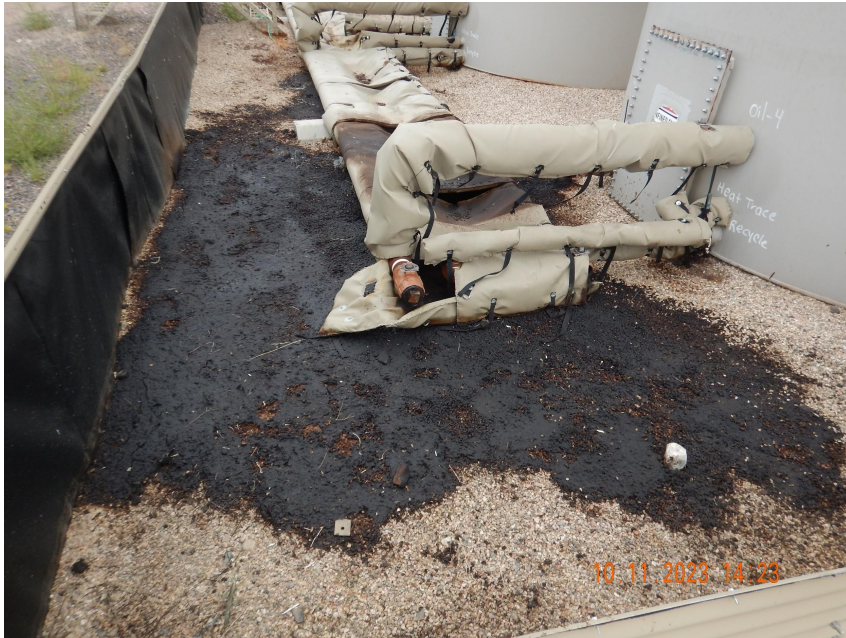
Photo 9. Photo taken from within the secondary containment. Stained soil/gravel needs to be removed, cleaned out and properly disposed of.
