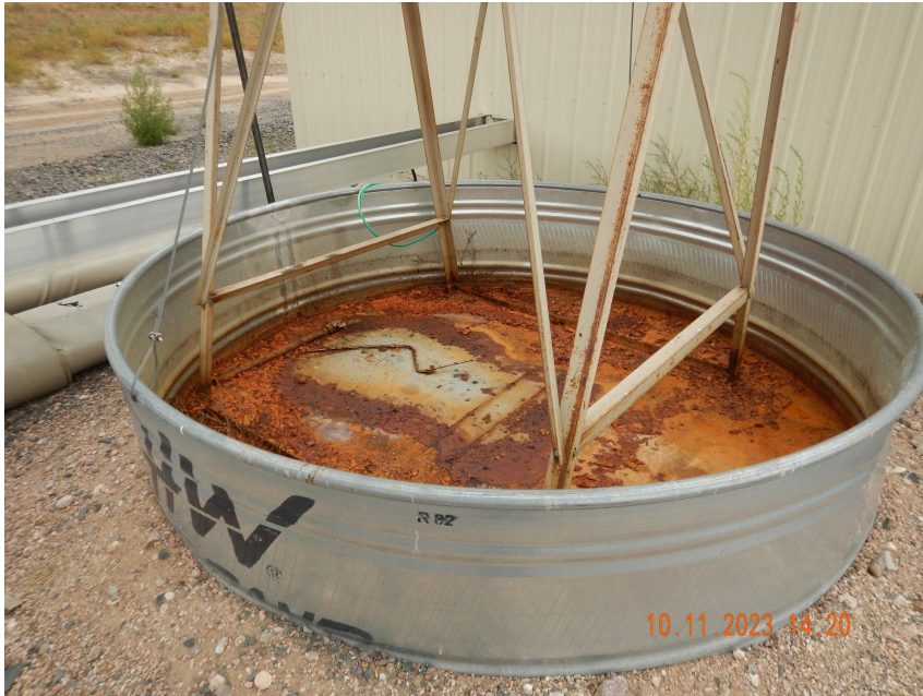
Photo 7. Photo taken of secondary containment which is missing wildlife protection (netting). Secondary containment is for coolant.
