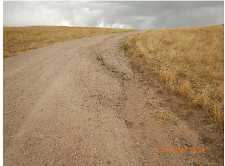
Photo 10. Photo taken along a portion of the access road, facing West. Photo illustrates rill erosion in need of repair.
