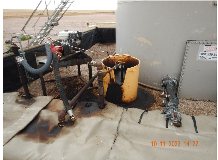
Photo 8. Photo taken from within the secondary containment. Stained soil/gravel needs to be removed, cleaned out and properly disposed of.
