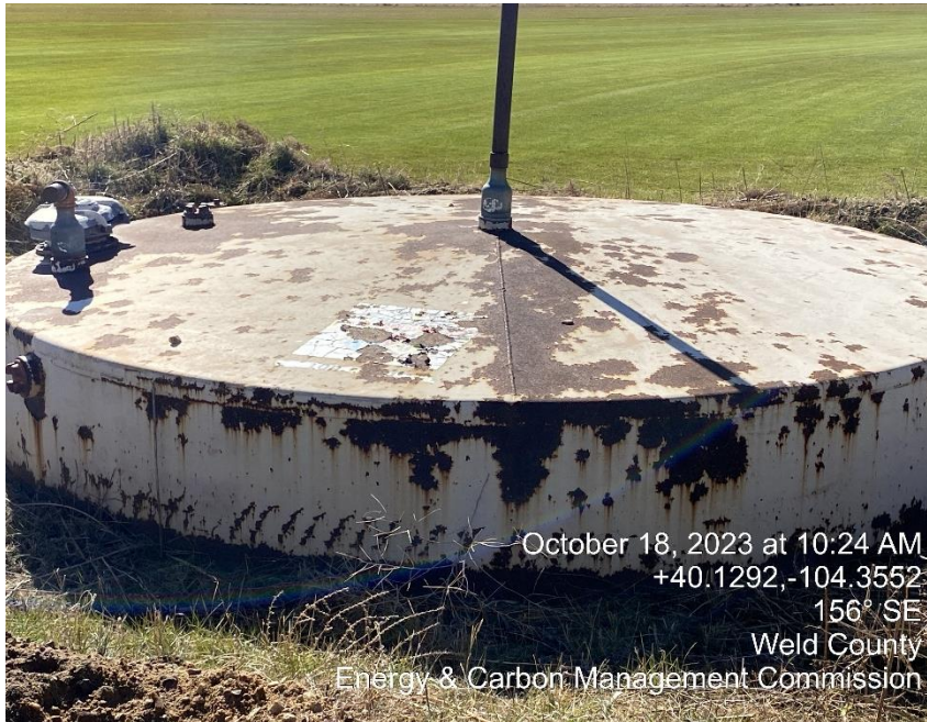
Missing Capacity/ NFPA Placard
