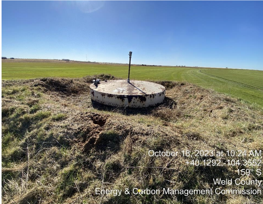
Removed Overgrown Vegetation & Missing Capacity/ NFPA Placard
