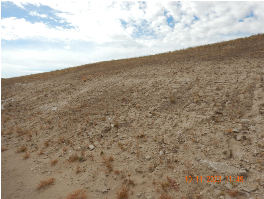
Photo 5. Photo taken from the western cut slope, facing West. Photo illustrates rill erosion is evident. Operator continues to try and seed the cut slope which is not sufficient.
