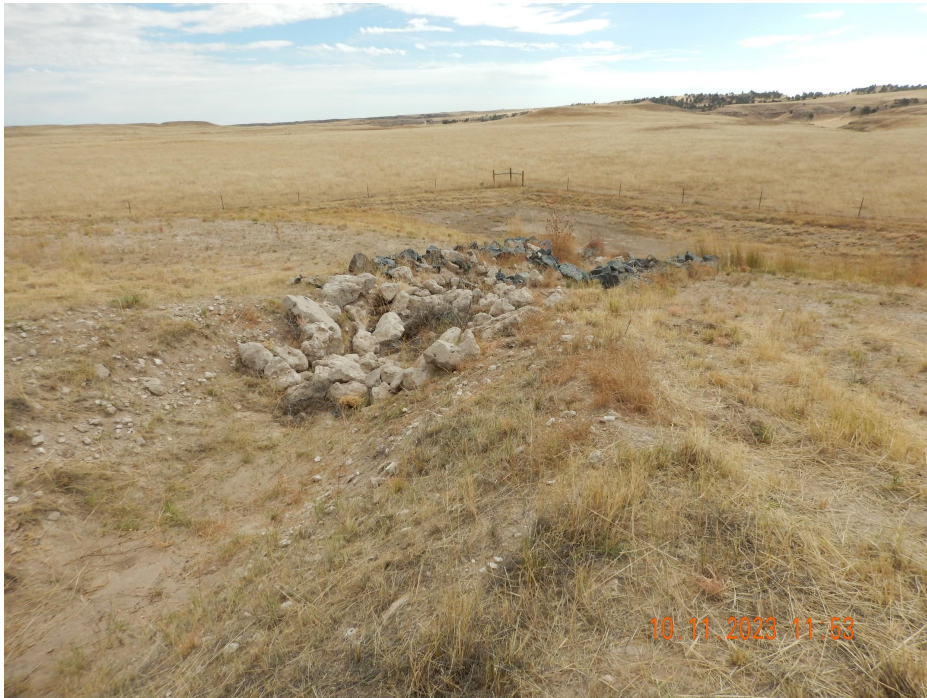
Photo 3. Photo taken from the southeastern interim area, facing Southeast. Photo illustrates the Operator has made stormwater erosion repairs.
