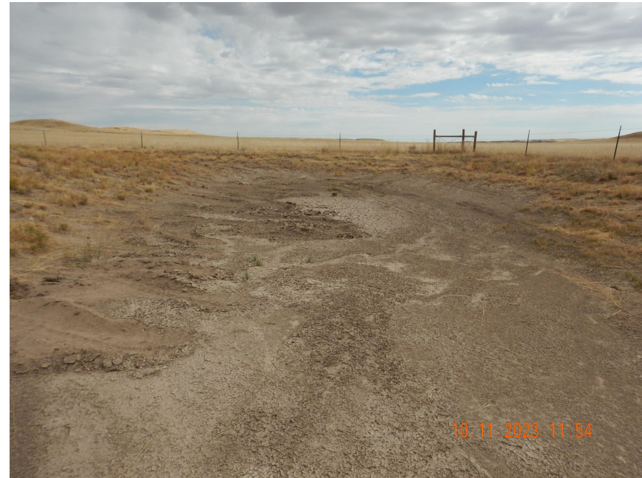
Photo 4. Photo taken from the southeastern interim area, facing East. Photo illustrates the retention pond is functioning properly and no observed sediment discharge from location.
