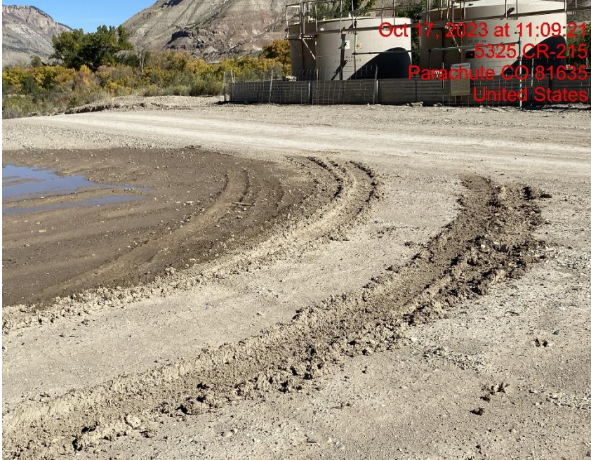
Lack of Stabilization/Insufficient Vehicle Tracking BMPs at Location Entrance/Exit – Photo #06980
