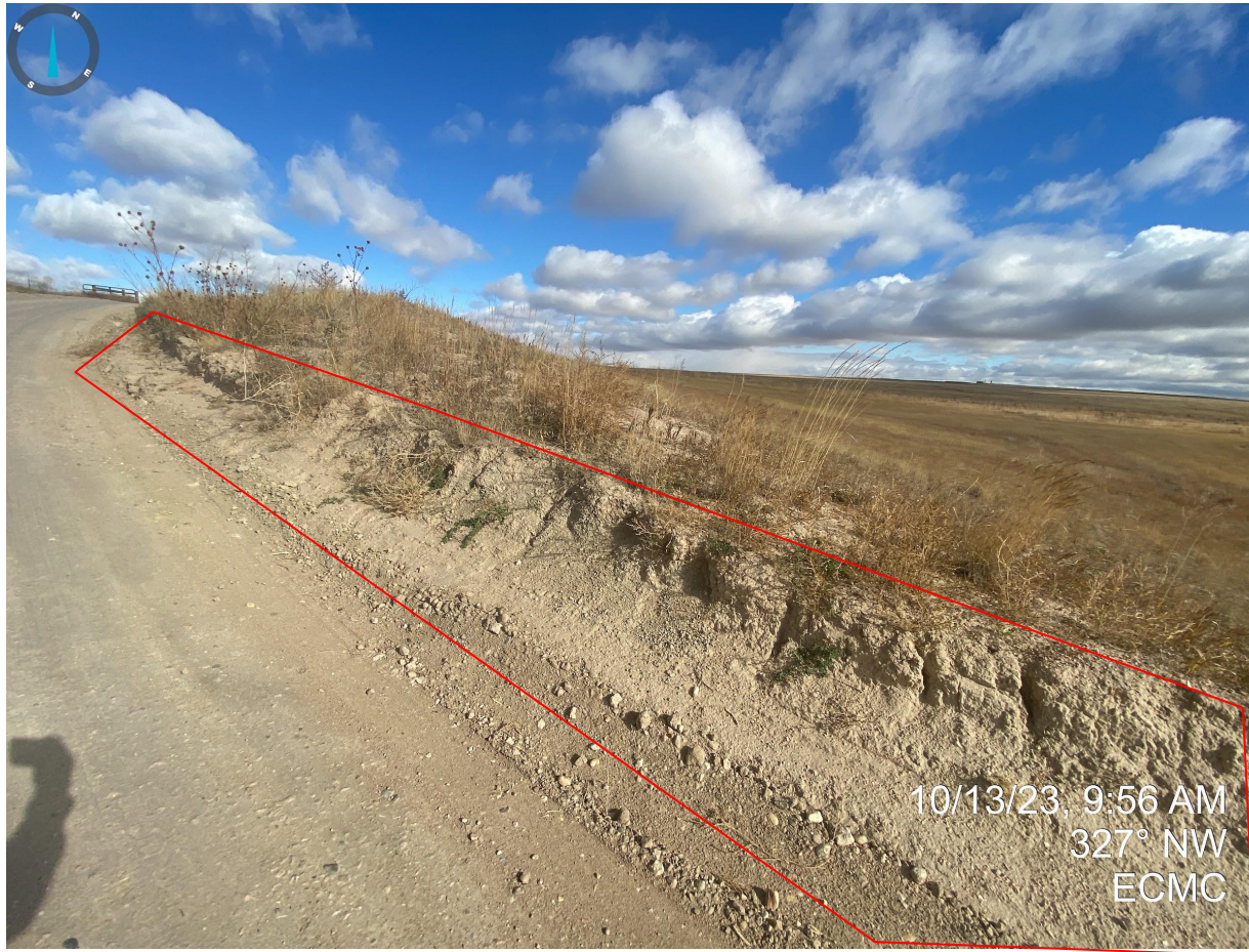
Photo 1. Taken from the access road. Photo illustrates unstabilized soils and evidence of erosion degradation.
