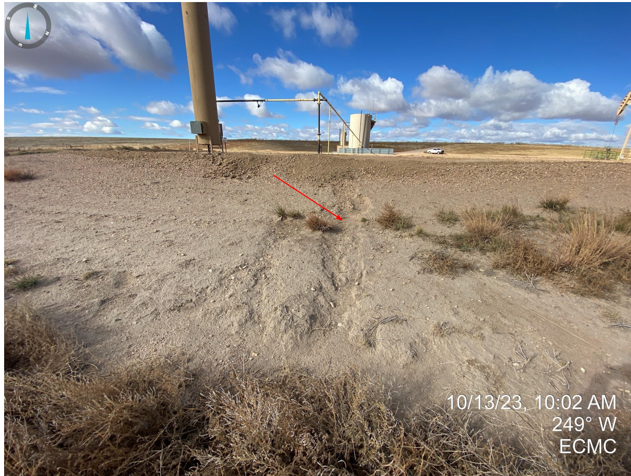
Photo 5. Unstabilized soils and erosion degradation on the east side of the location.
