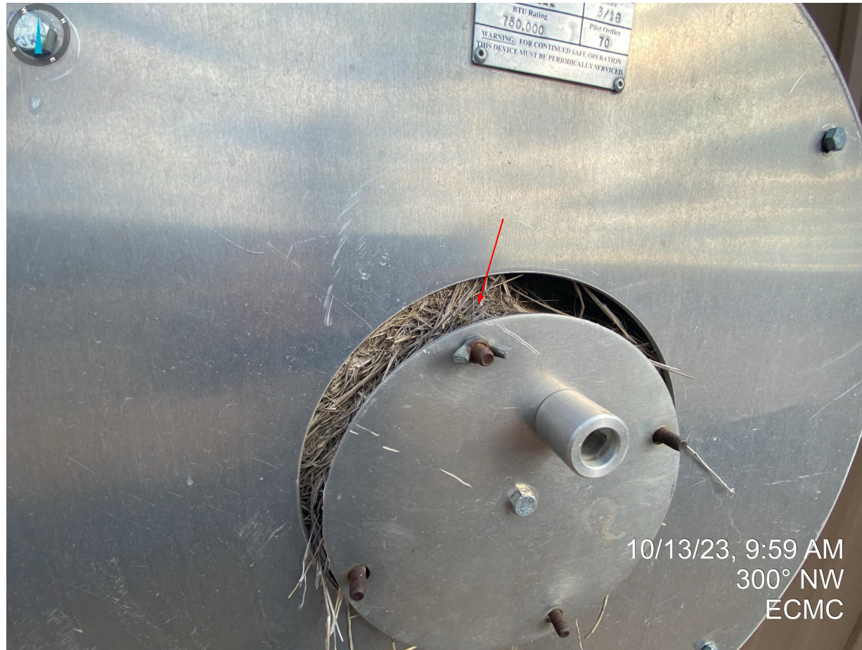
Photo 9. Bird nest within vertical separator and absence of wildlife exclusion device.
