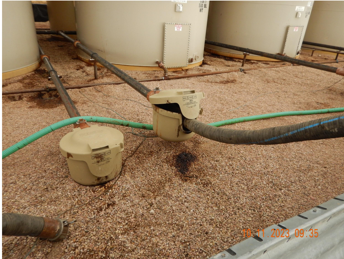
Photo 3. Photo taken from the secondary containment area. Photo illustrates stained soil that needs to be cleaned up and removed. Also, load out lines were observed being stored inside secondary containment. This would be considered unused equipment.
