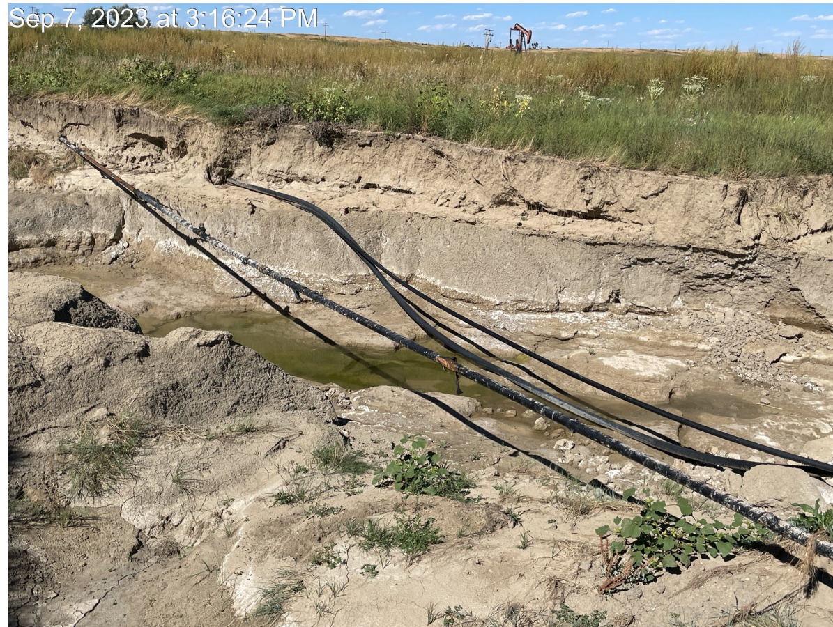
Photo 10. Photo taken facing north, of large gully with exposed un-stabilized flowlines
