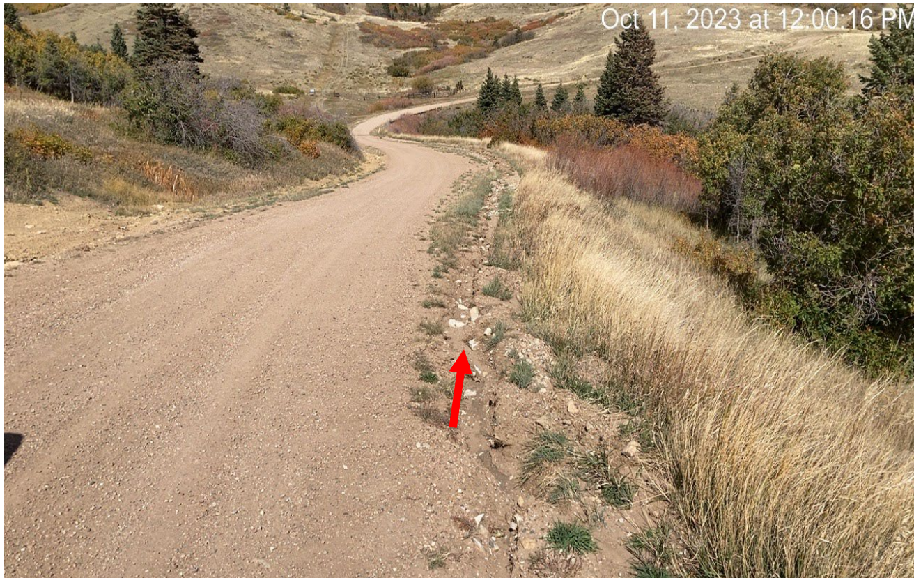
Photo 3. Facing northwest back down the access road. Grading has pushed out material into a berm which is not allowing stormwater to be diverted off the road. There is a long stretch of the road where stormwater will be directed down the road which will cause erosion.
