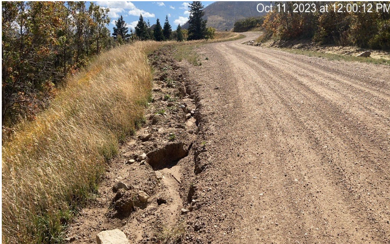
Photo 2. Facing southeast along the east side of the road. Grading has pushed out material into a berm which is not allowing stormwater to be diverted off the road.
