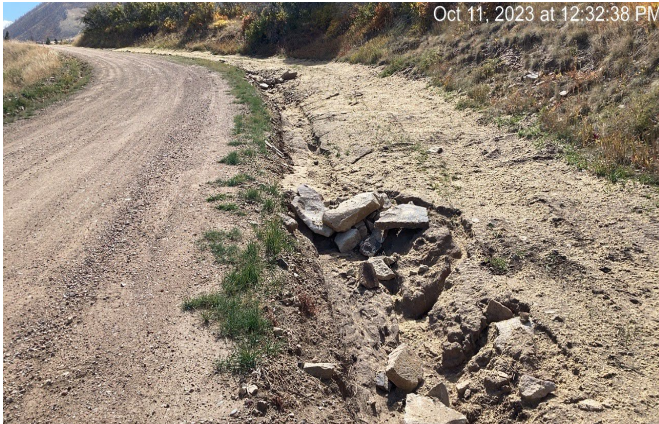
Photo 4. Facing southeast along the east side of the road. Some of the rock check dams installed have filled in with sediment and need maintenance. There was erosion observed underneath some of the rocks which were not properly constructed.
