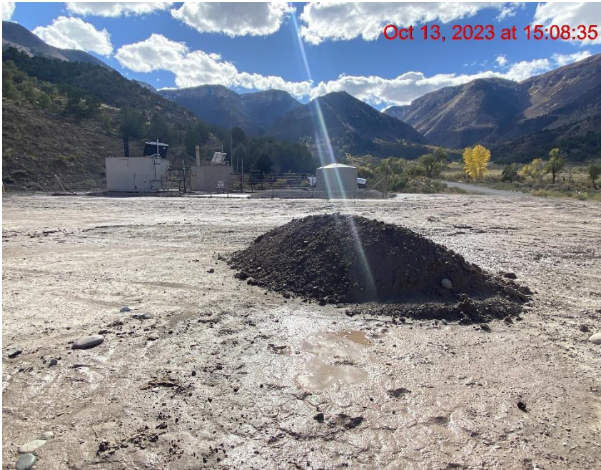
Unprotected Soil Stockpile – Photo #06921
