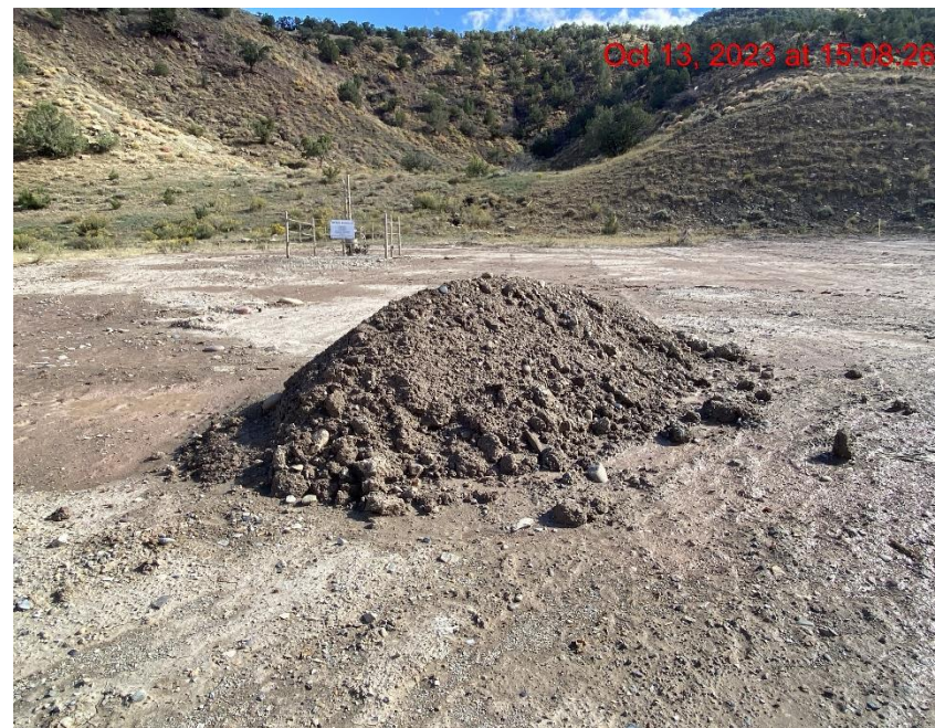
Unprotected Soil Stockpile – Photo #06920
