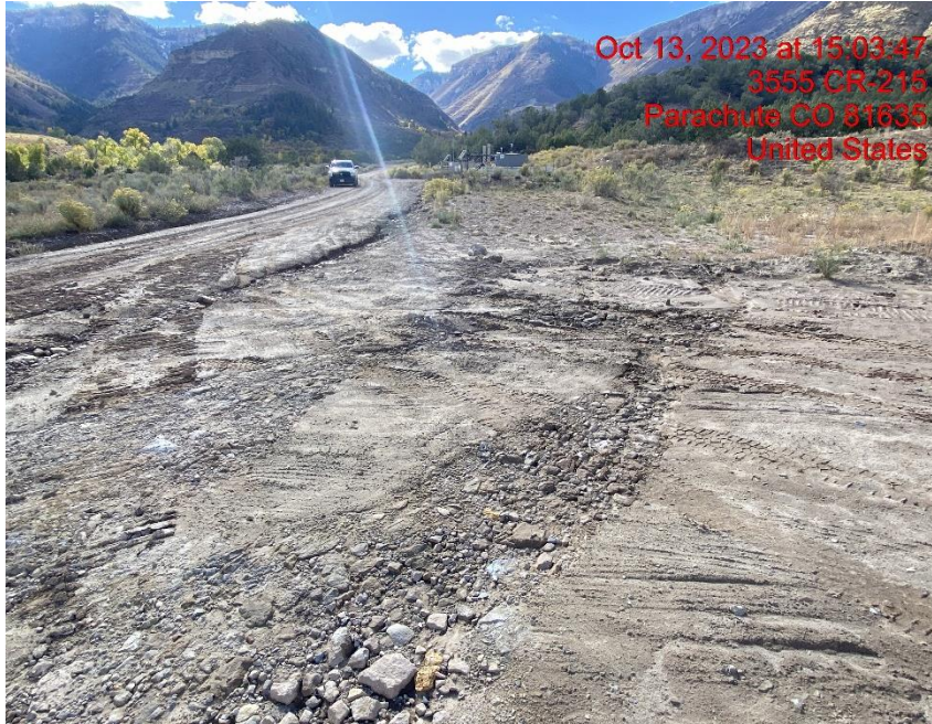
Lack of Stabilization/Insufficient Vehicle Tracking BMPs – Photo #06913
