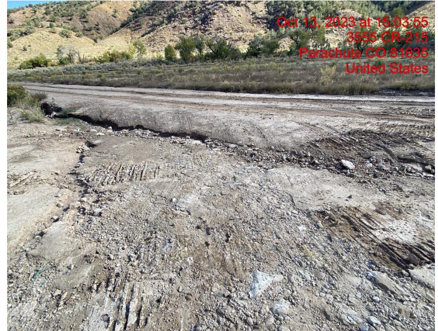
Lack of Stabilization/Insufficient Vehicle Tracking BMPs – Photo #06914
